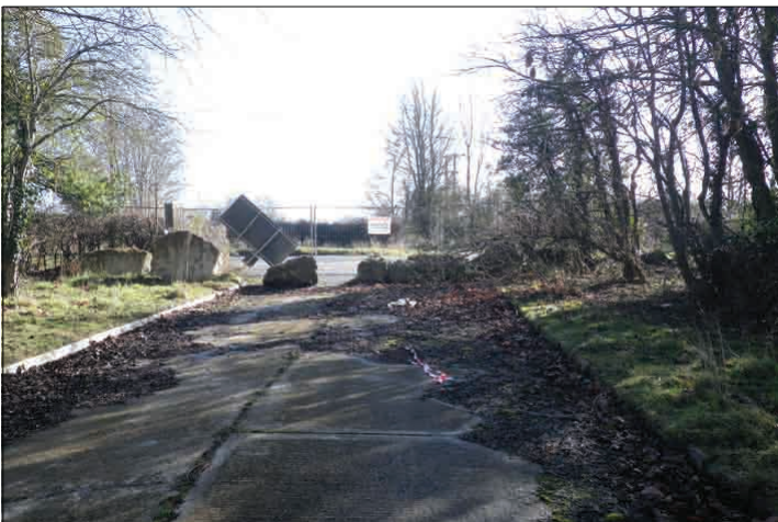
Plate 3 View from west showing a former entrance into the Cement Works from Haslingfield Road, with Railway tracks and screening bank (on right)
