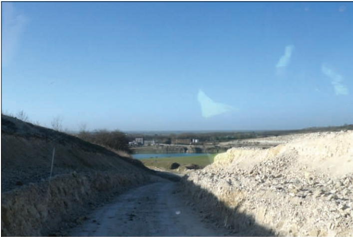
← Plate 5 View of water-filled quarry (Zone 2) and Cement Works (Zone 1) taken from track leading down from the Old Barrington Chalk Pit
