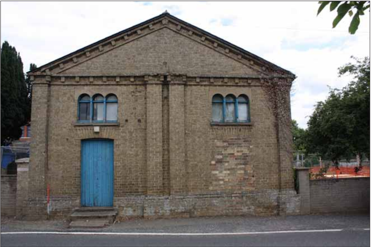
Plate 7: West-facing elevation (taken from High Street)
