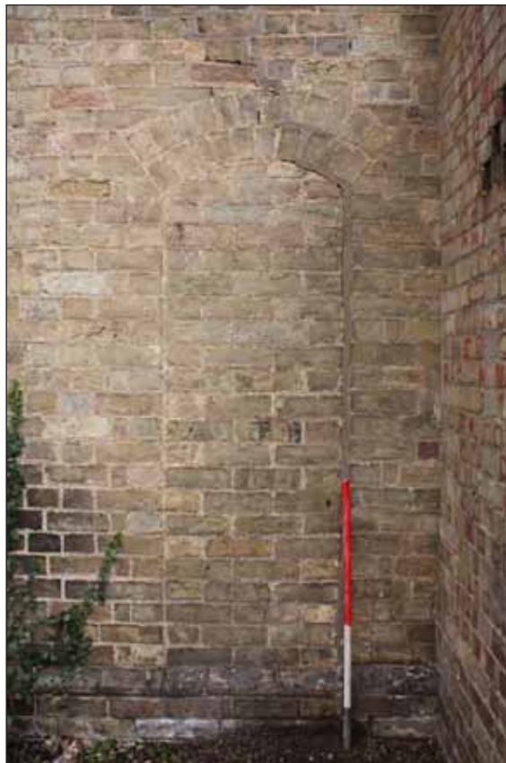
Plate 6: Blocked doorway, south-facing elevation
