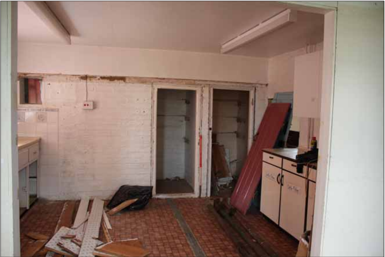
Plate 21: Detail of inserted cupboards room 2
