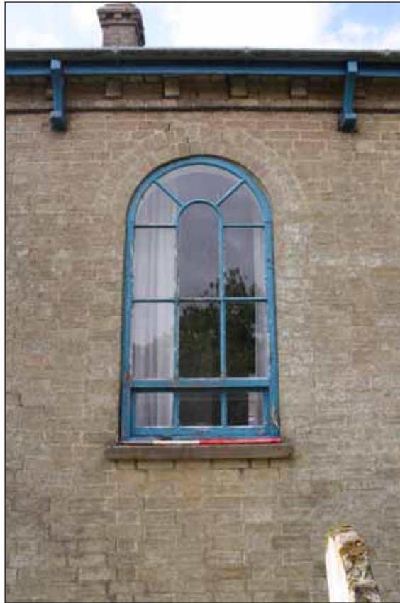
Plate 3: Detail of arched window, north facing elevation
