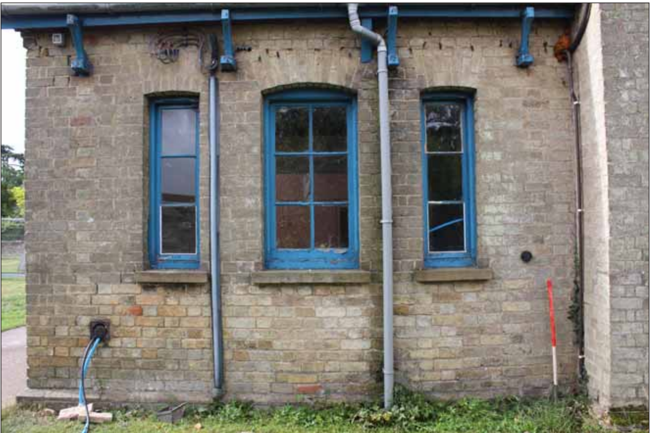
Plate 2: Fenestration on eastern extension, north facing elevation
