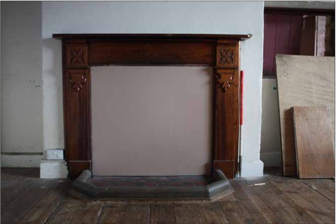
Plate 19: Detail of fireplace at eastern end of main hall
