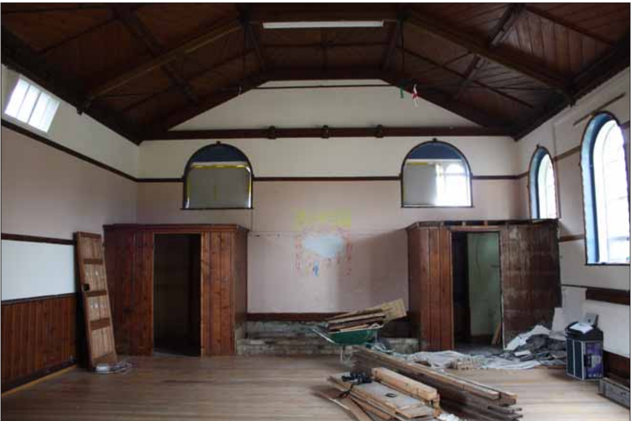
Plate 14: Mail hall (R1) entrance "rooms"
