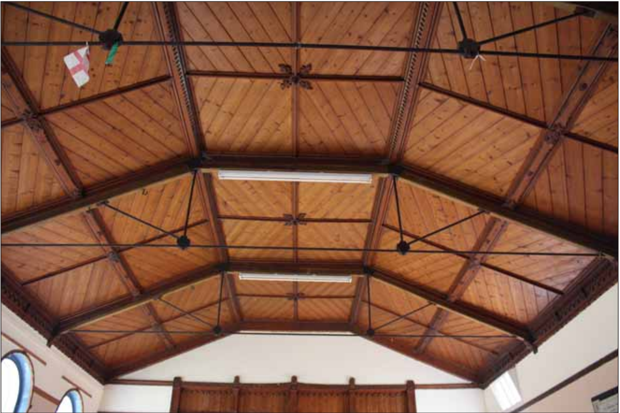
Plate 13: Detail of ceiling
