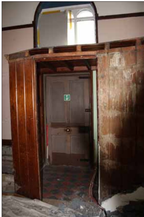
Plate 16: Entrance room on right-hand side
