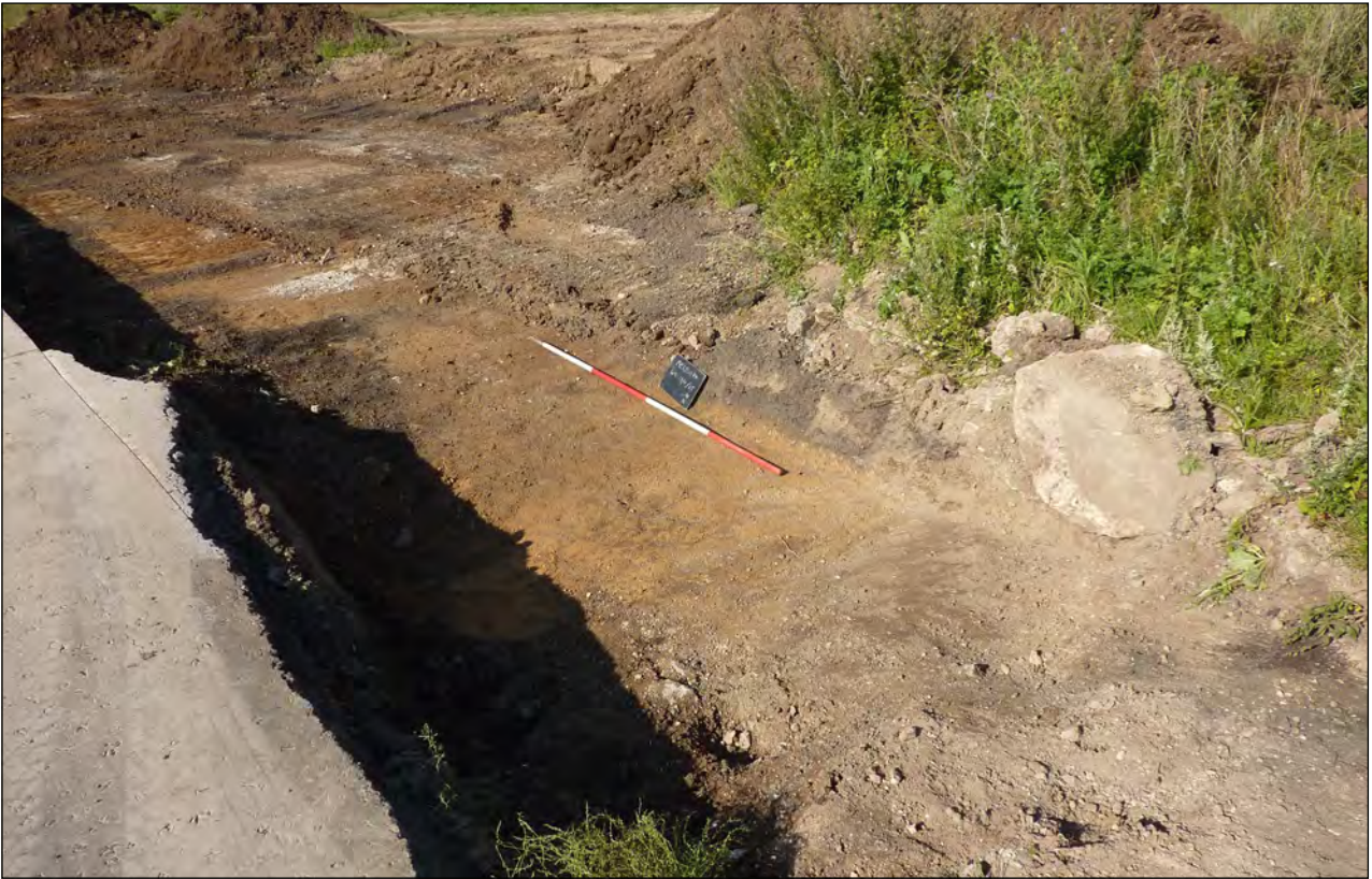
Plate 13: Scheduled area following removal of access road material. View northwest.
