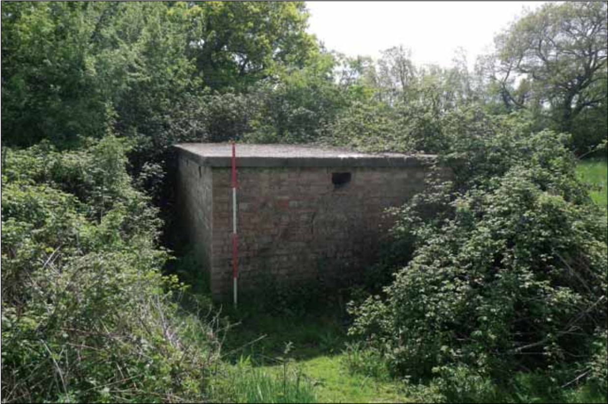
Plate 1: Home Guard Store in Field 1, facing south
