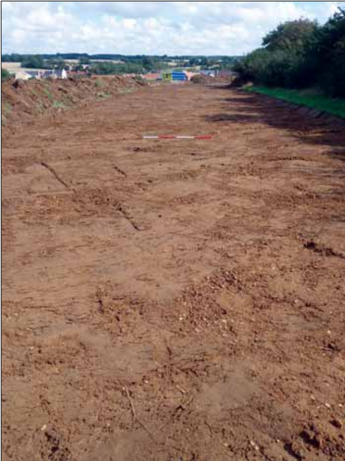
Plate 1: Site conditions between chainage 500m and 750m, facing north-east
