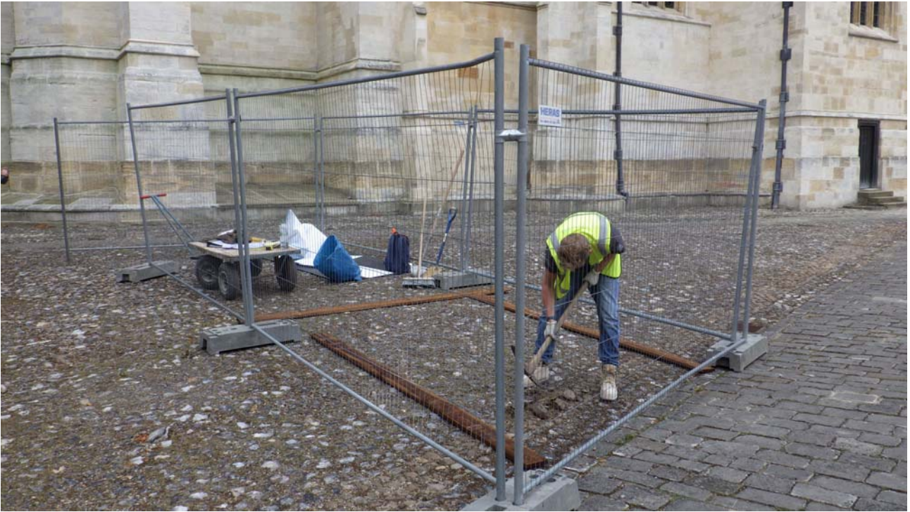
Plate 3: Hand excavation of the cobbles within Trial Area B
