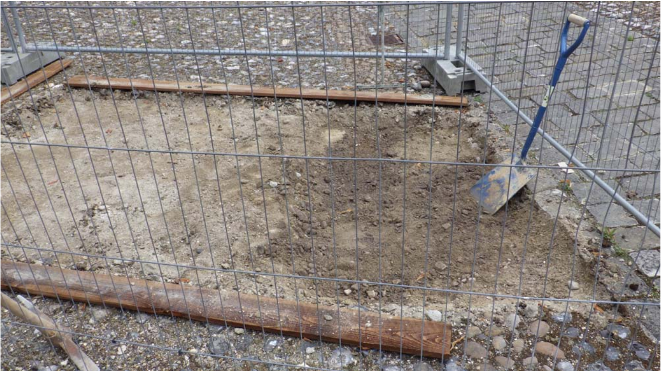
Plate 8: Excavated surface Trial Area C
