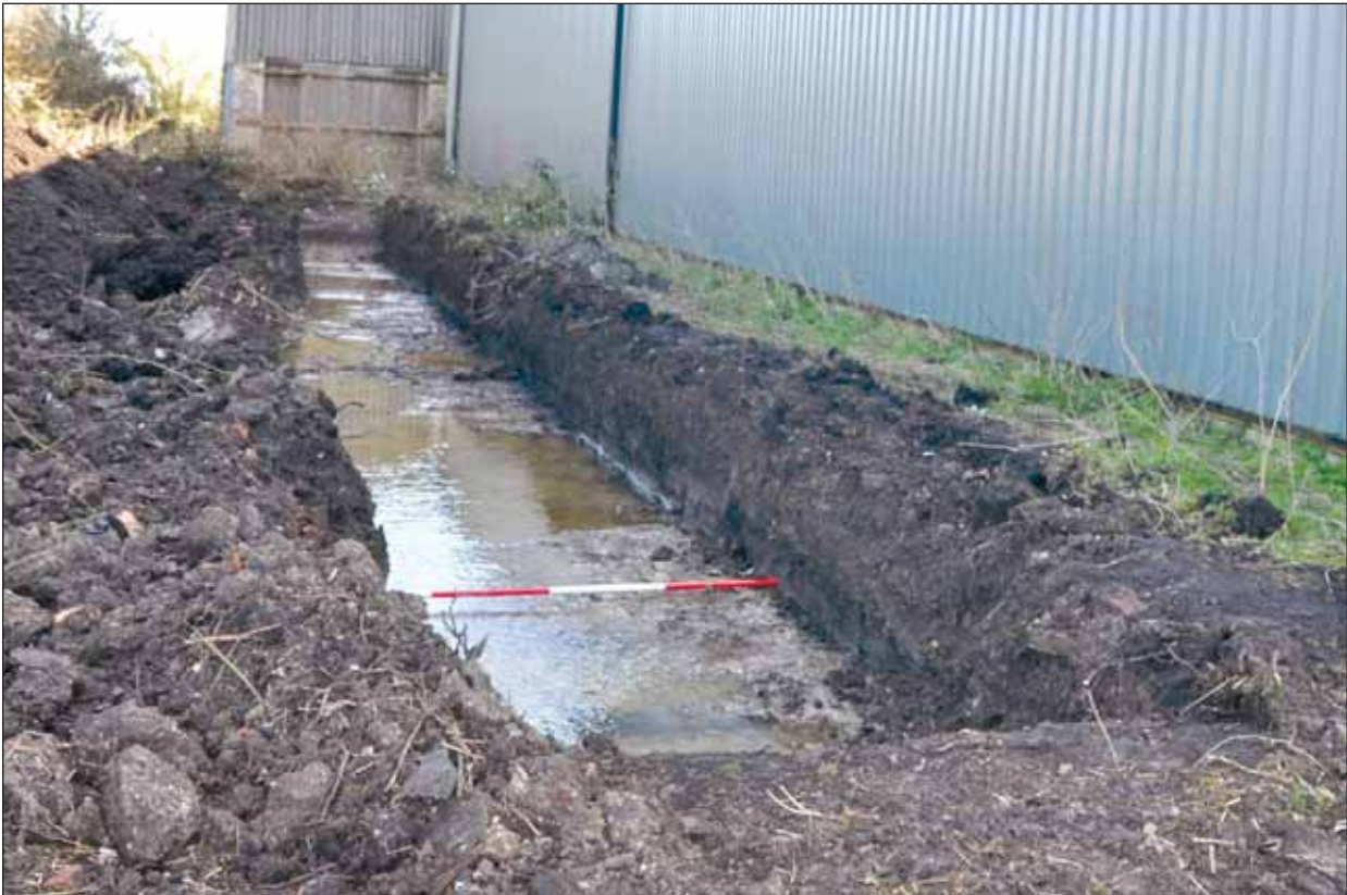
Plate 1: General view of Trench 1, viewed from the north-west
