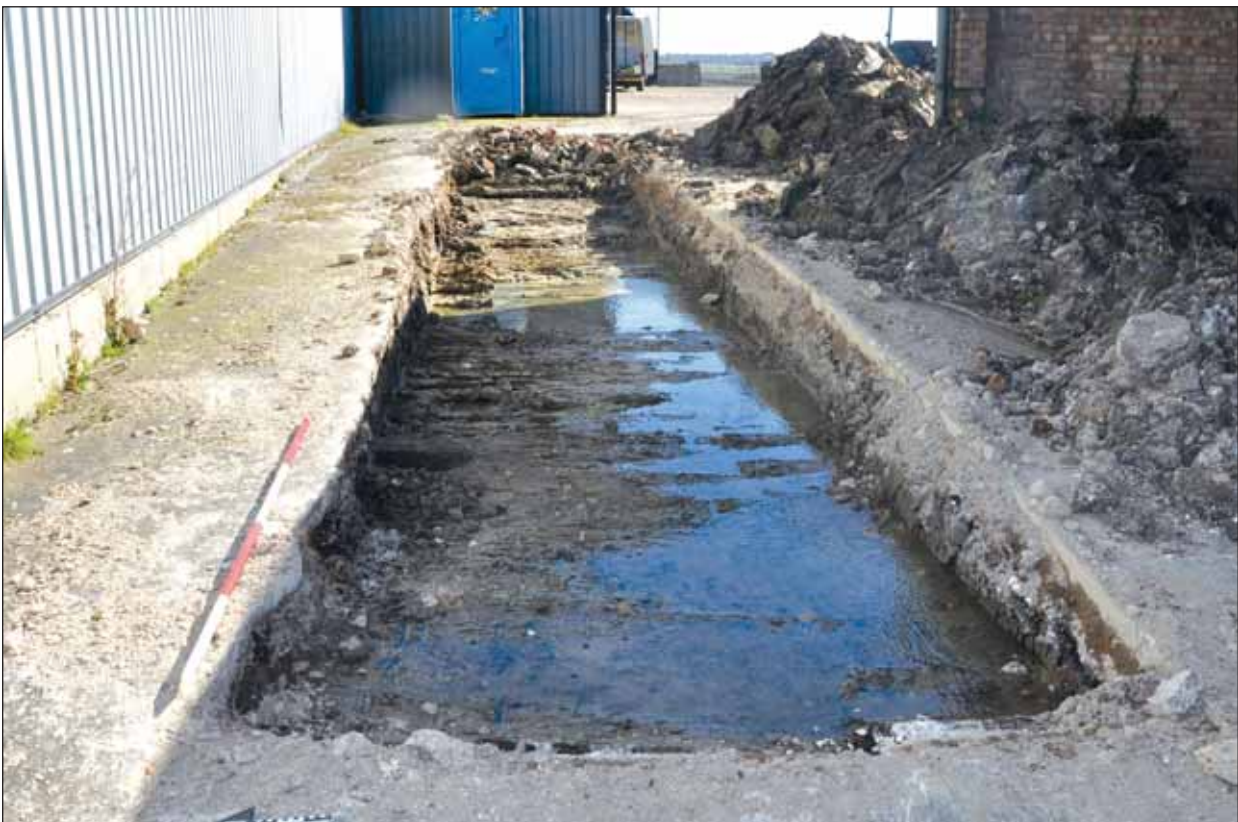
Plate 4: Trench 3, viewed from the west showing its position between barns
