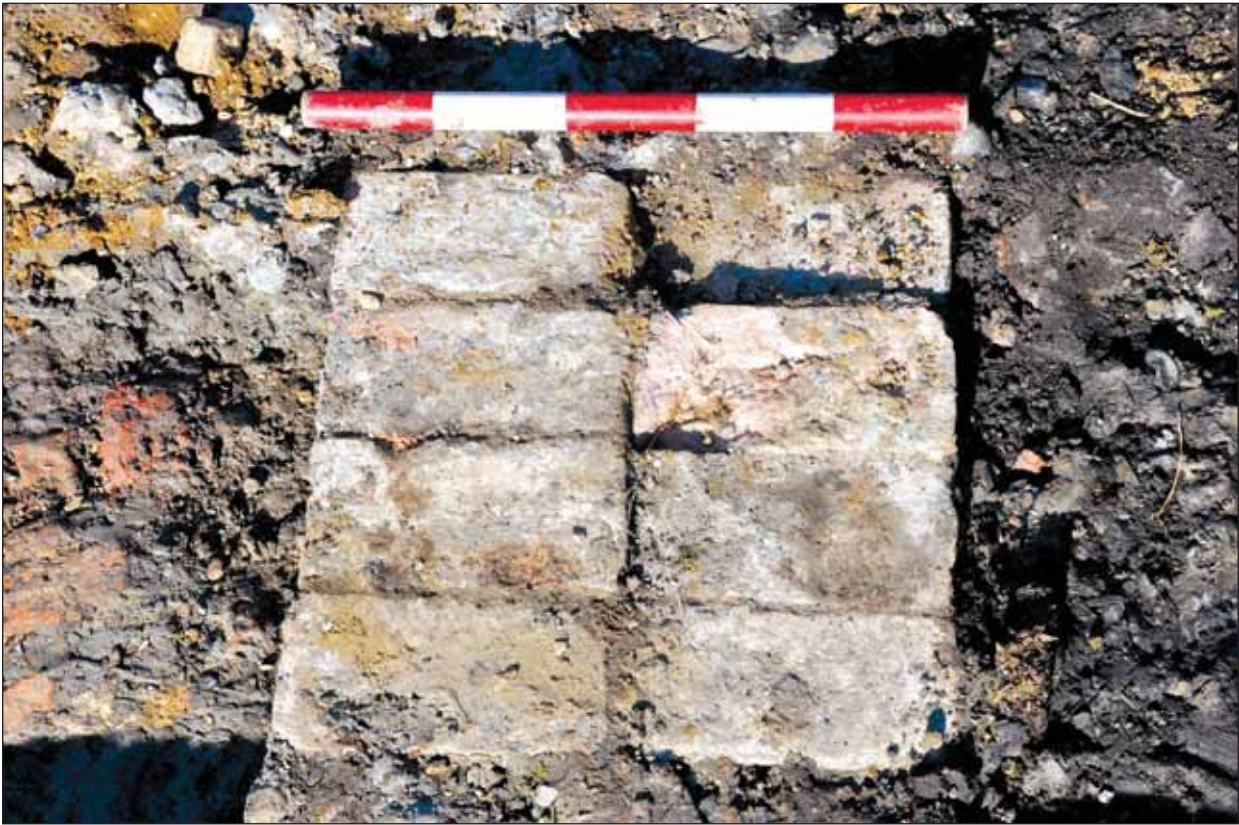
Plate 11: Trench 5, detail of brick foundation 505 , viewed from the south
