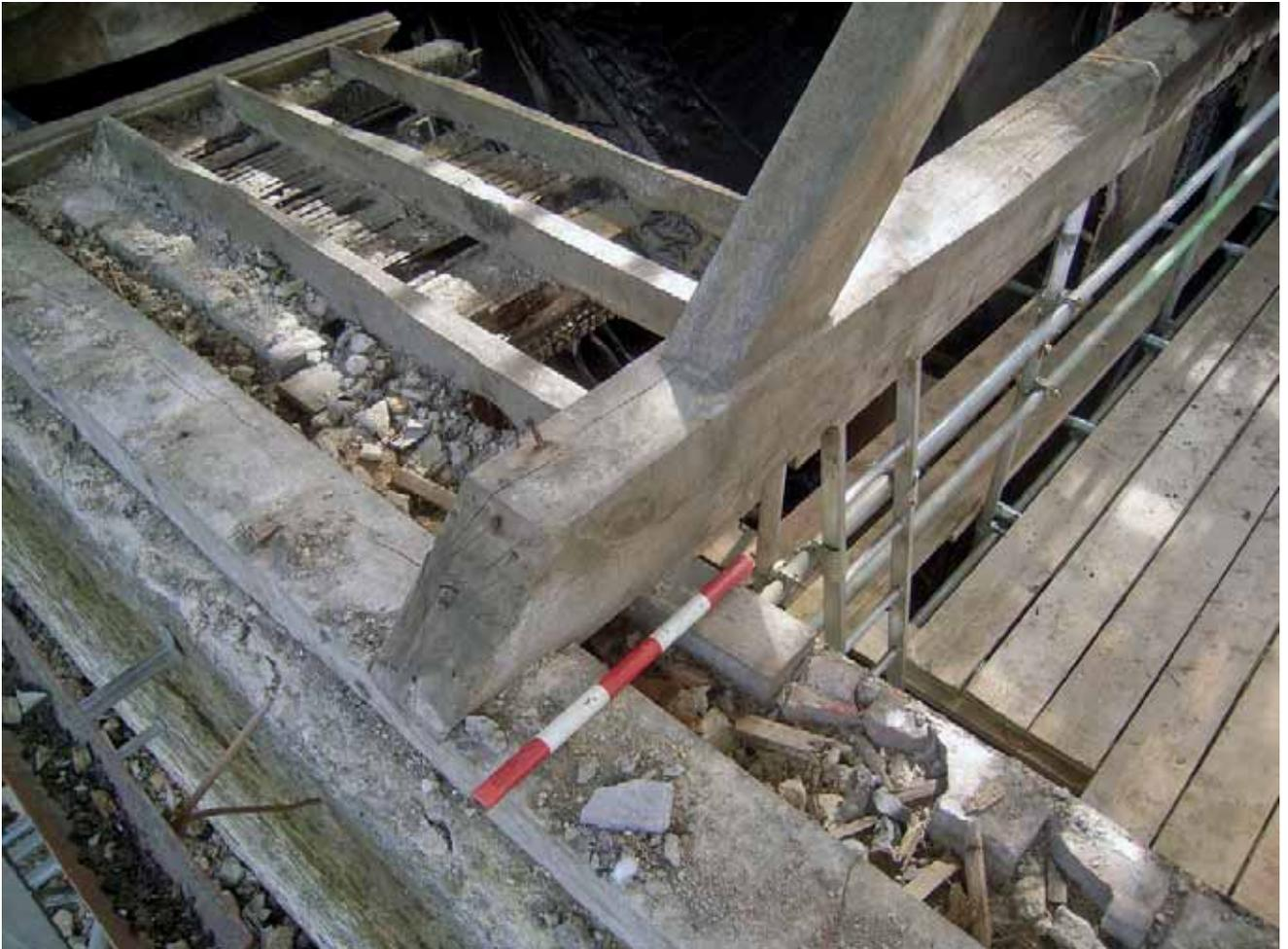
Plate 75: End of tie-beam in F1
