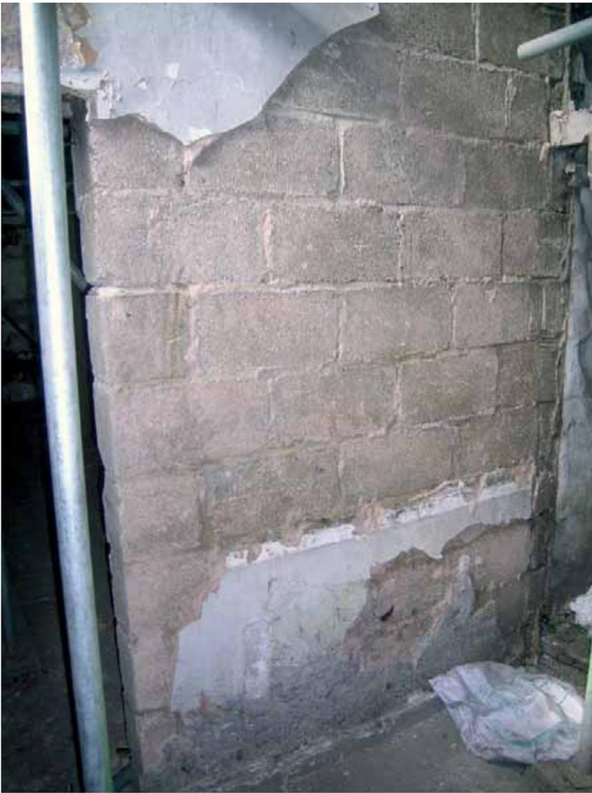
Plate 46: Concrete blockwork forming west wall of G4
