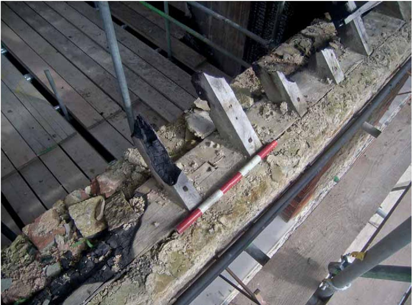
Plate 73: Wall plate with rafter feet in F1
