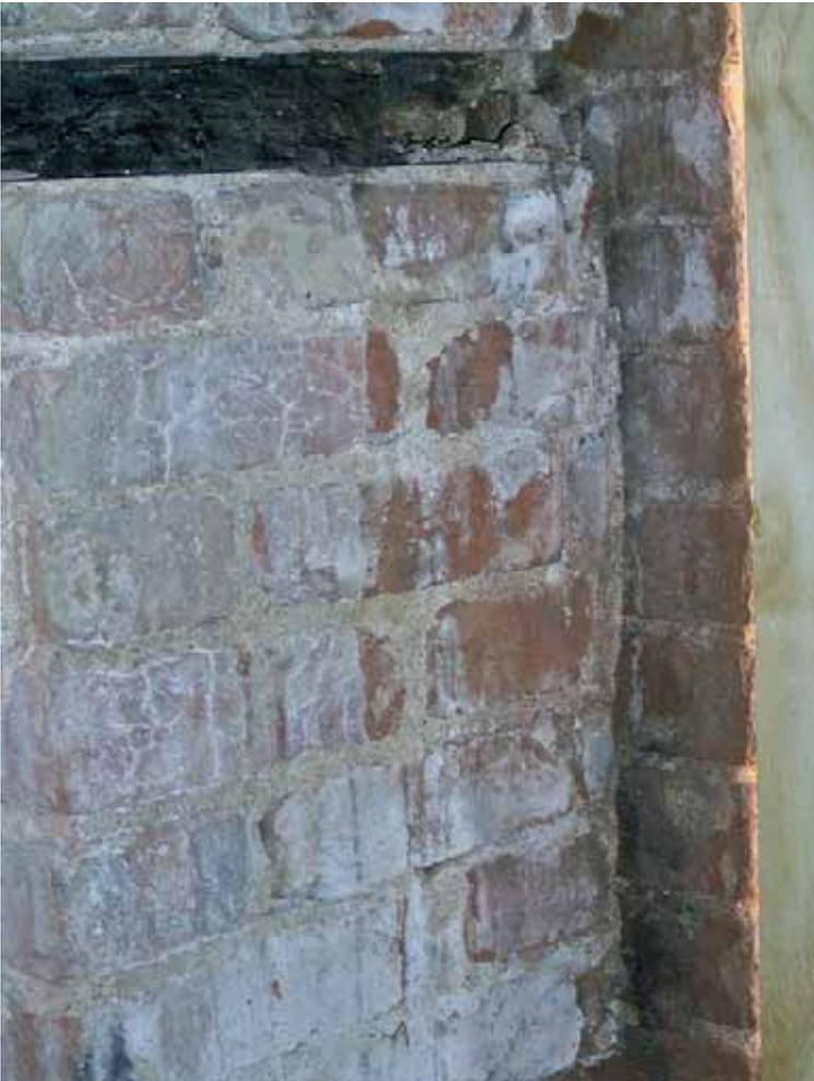
Plate 38: Jamb of window in G3 showing brick courses not aligning
