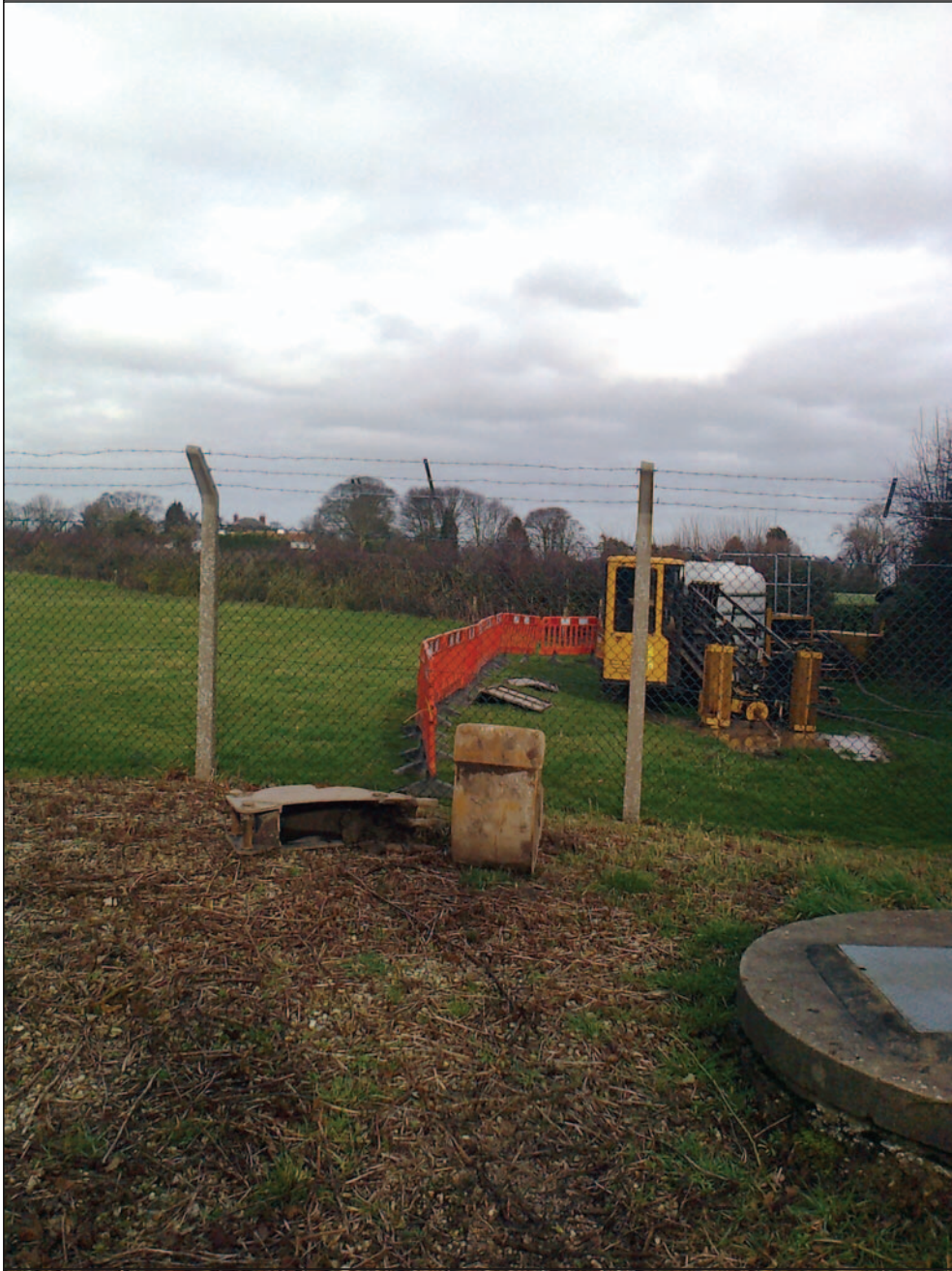
Plate 4: Work under way in Earthwork Field.
