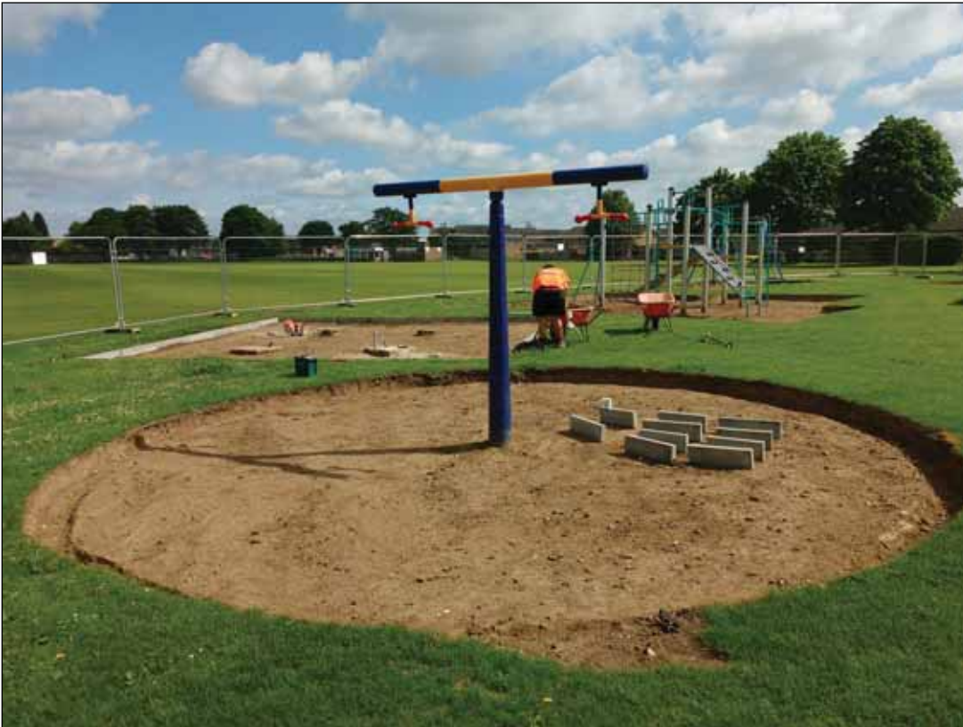
Plate 1: Soil strip around play equipment to north
