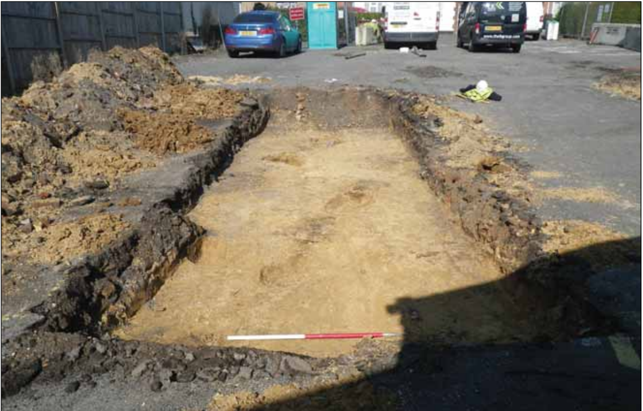
Plate 1: Trench 1, view north-northeast
