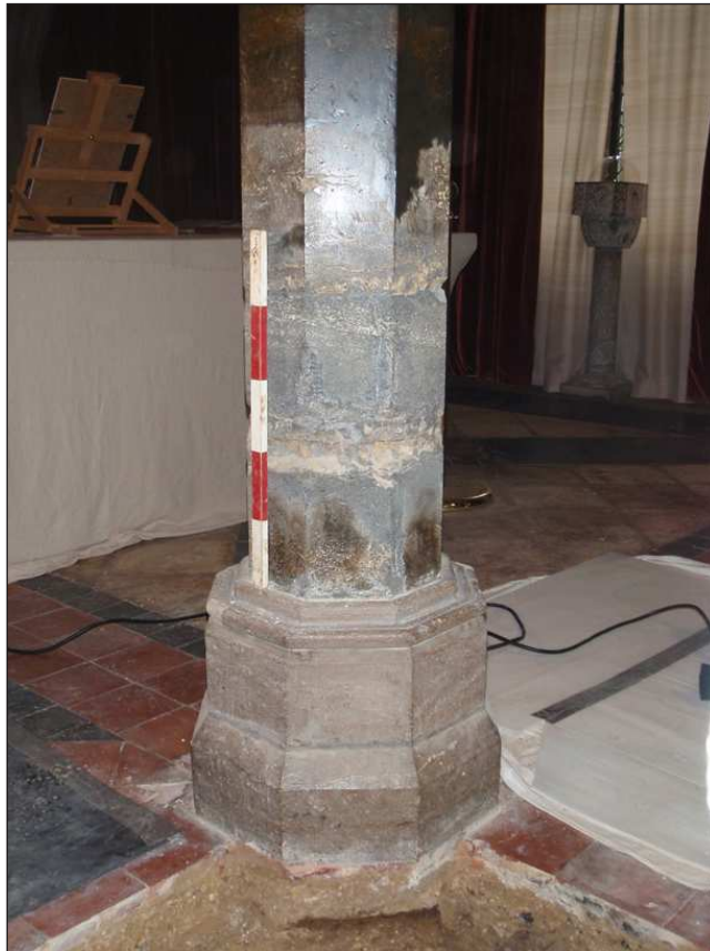
Plate 1: Column under investigation within dining room
