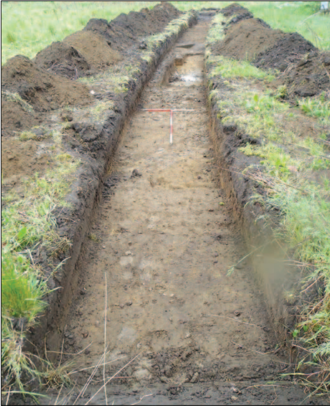
Plate 3: Trench 5, looking north-west
