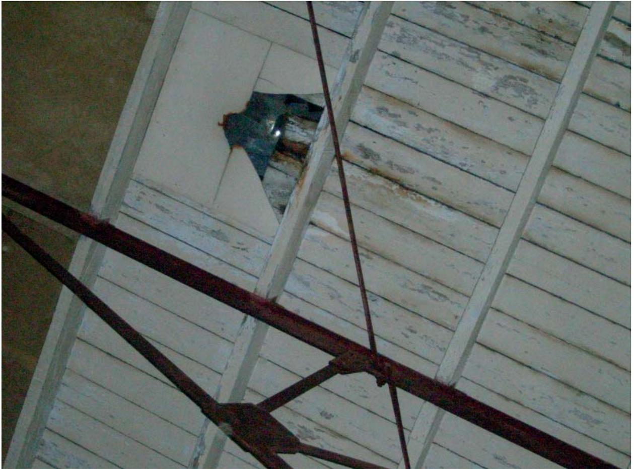
Plate 35: Detail of hole in roof from possible former flue
