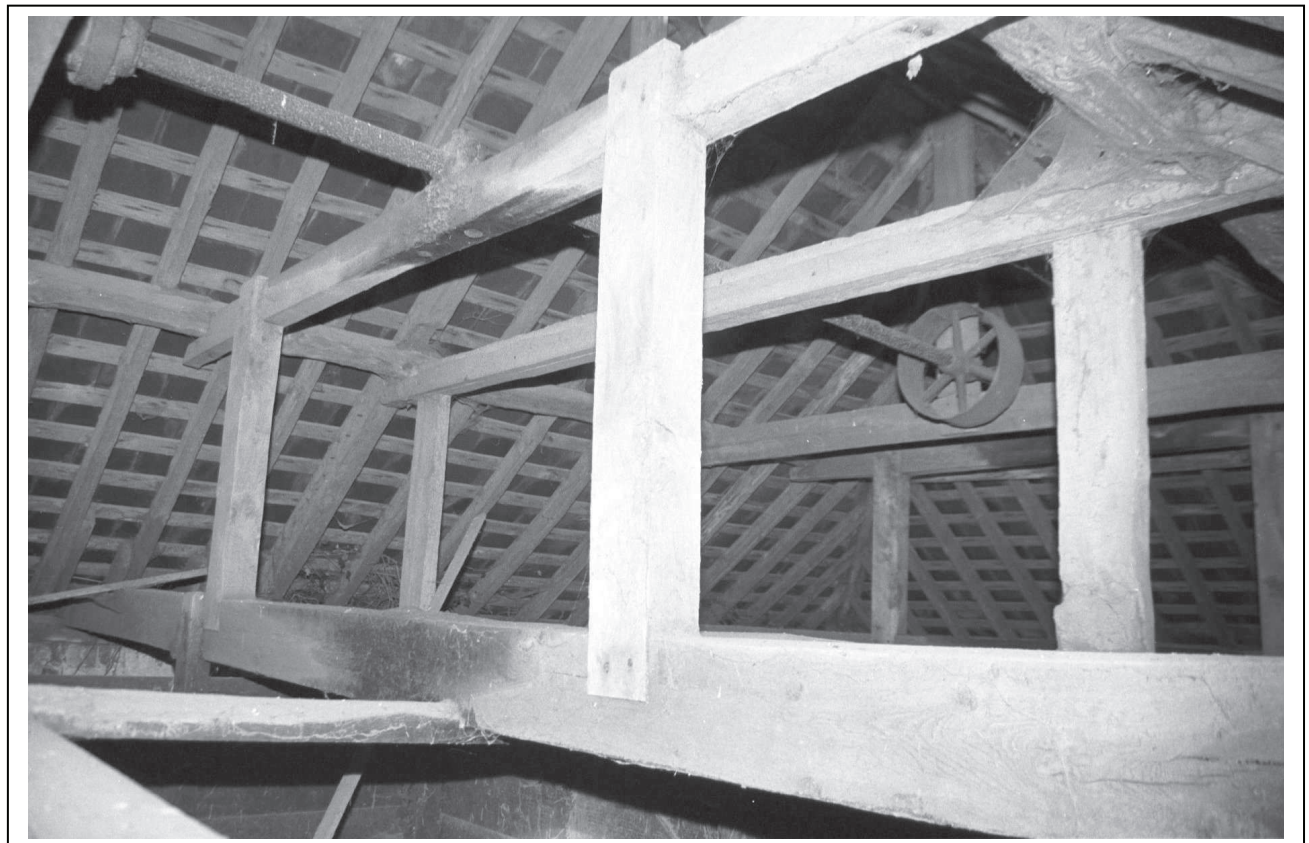
Plate 12: Power shaft and roof structure within wheel house. Looking towards south-east.
