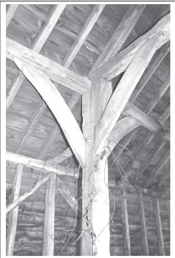
Plate 5: Truss 7 post detail
