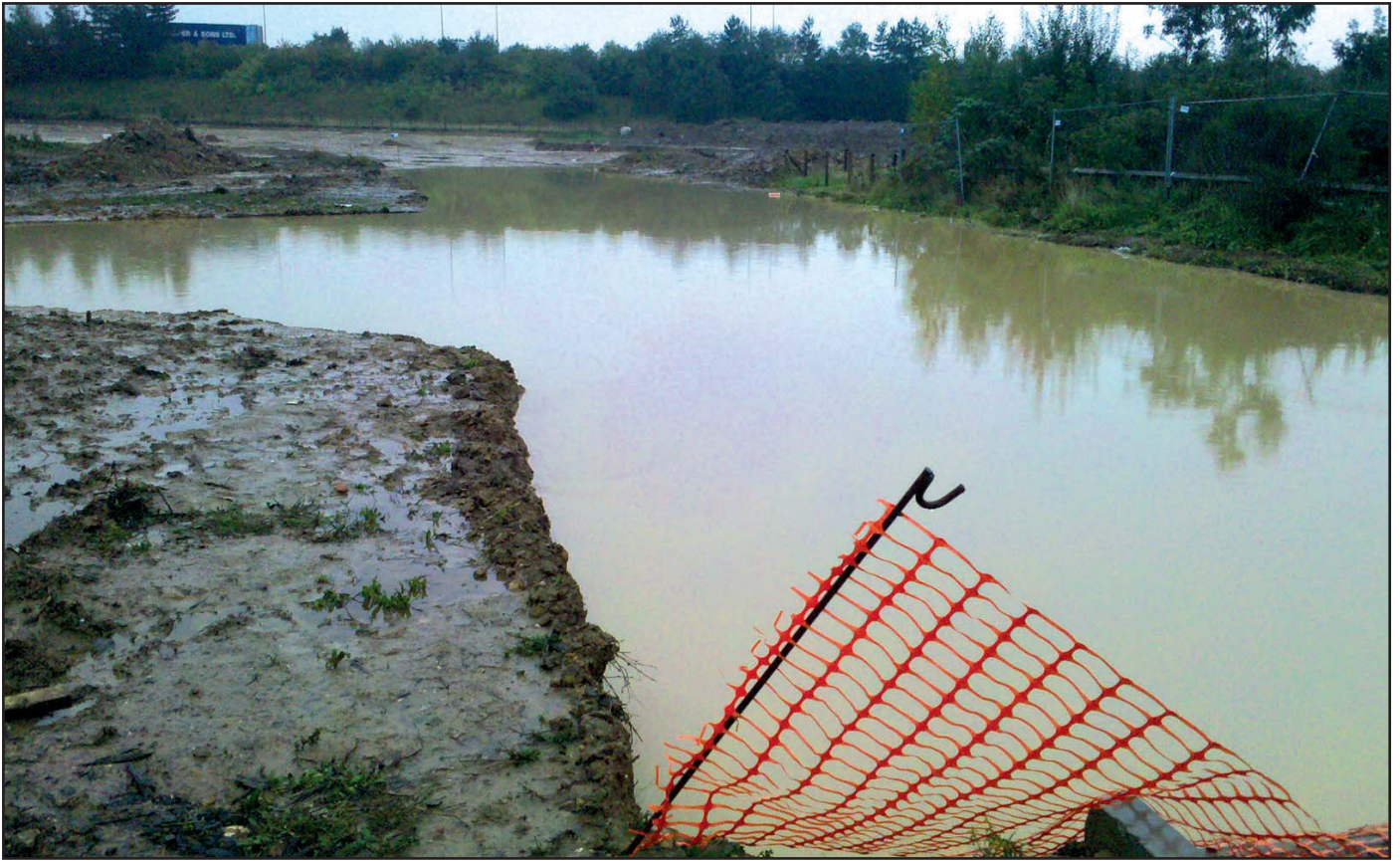
Plate 1: Flooding on site
