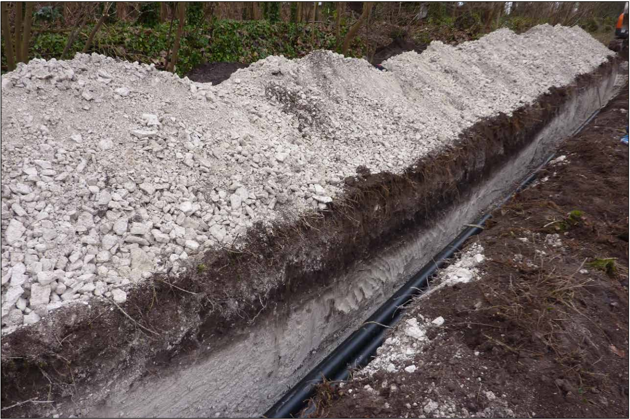
Plate 7: Hollow 140, Royston Road, view southwest
