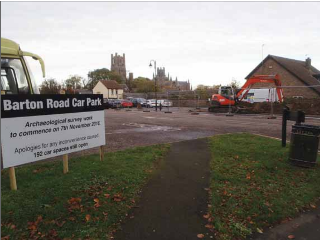
Plate 4: Working shot of Trench 1
