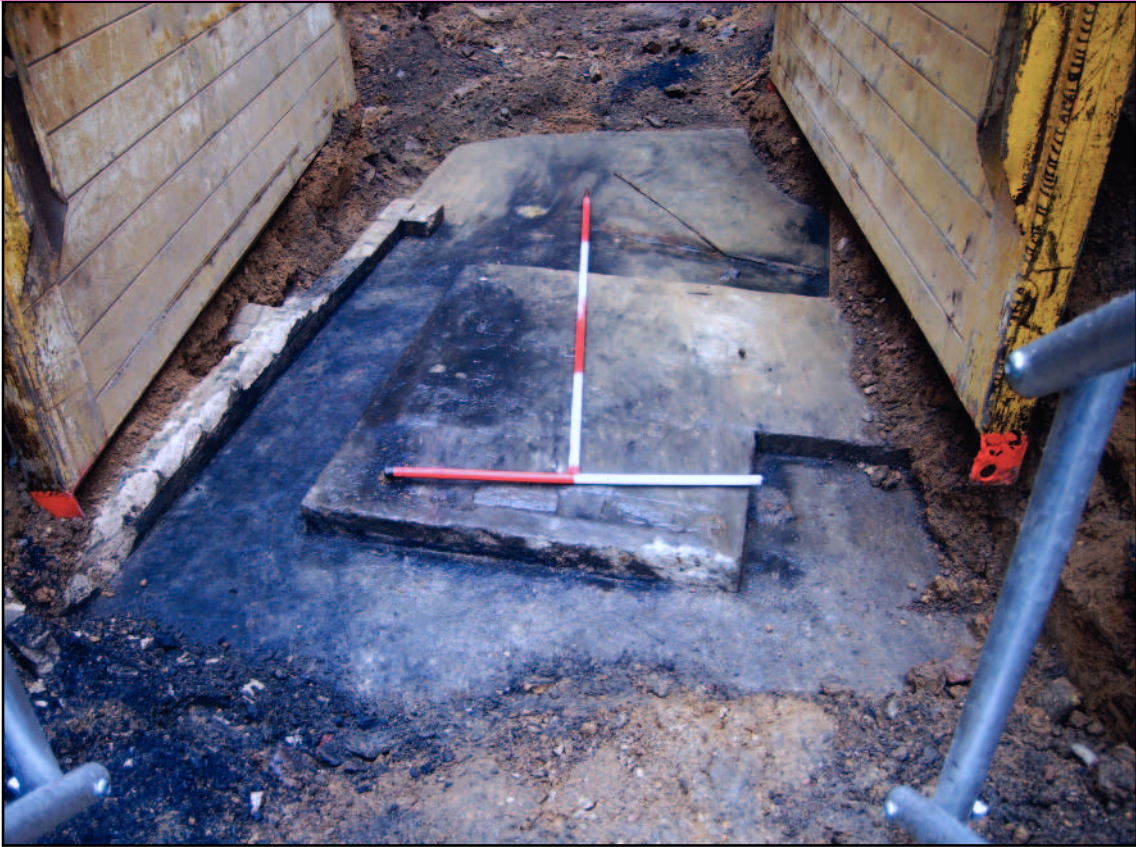
Plate 3: Concrete floor 206 in Trench 2, looking south.
