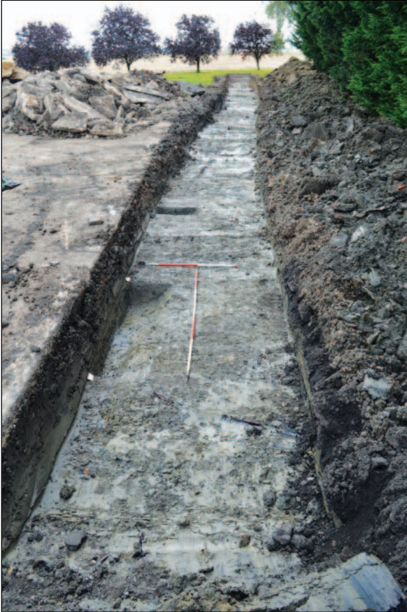
Plate 1: Trench 1, viewed from the north-east
