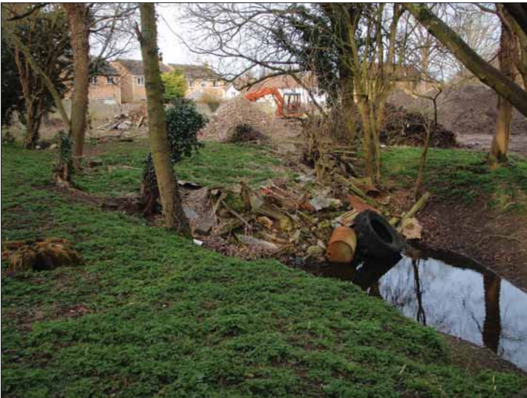
Plate 4: Western arm before works, viewed from west
