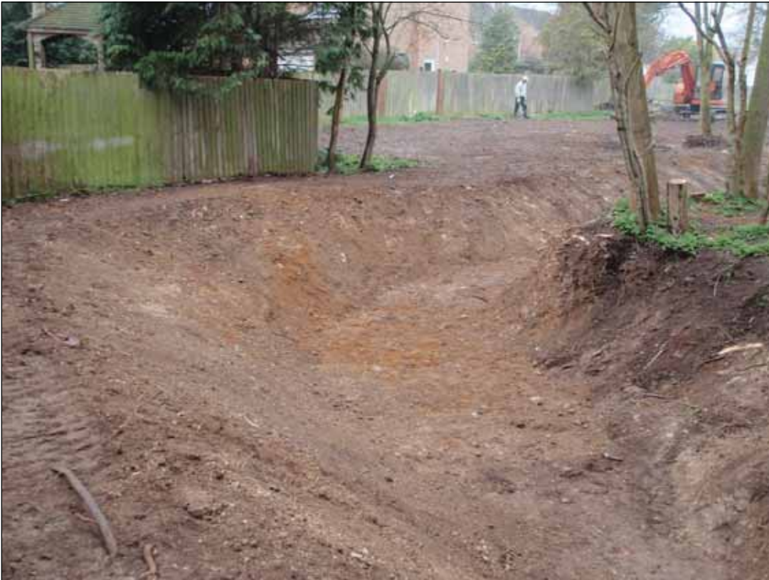
Plate 3: South-eastern corner after works, viewed from south-west
