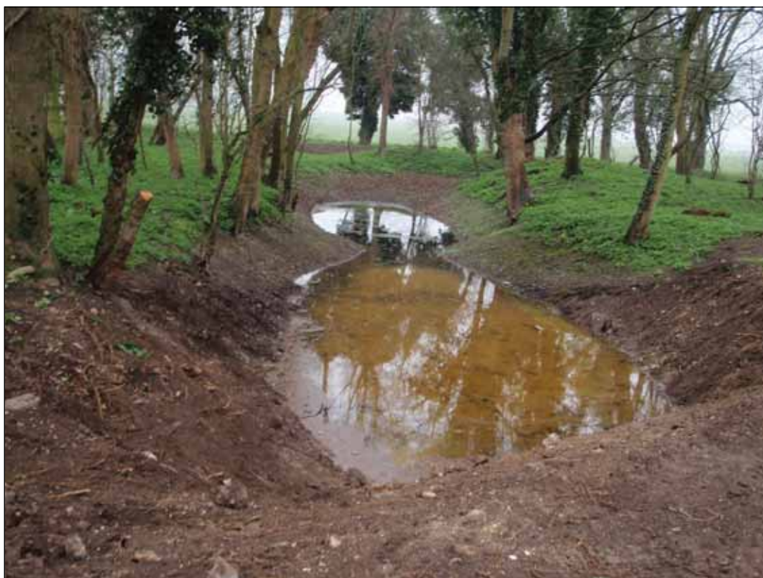
Plate 1: Northern arm after works, viewed from east
