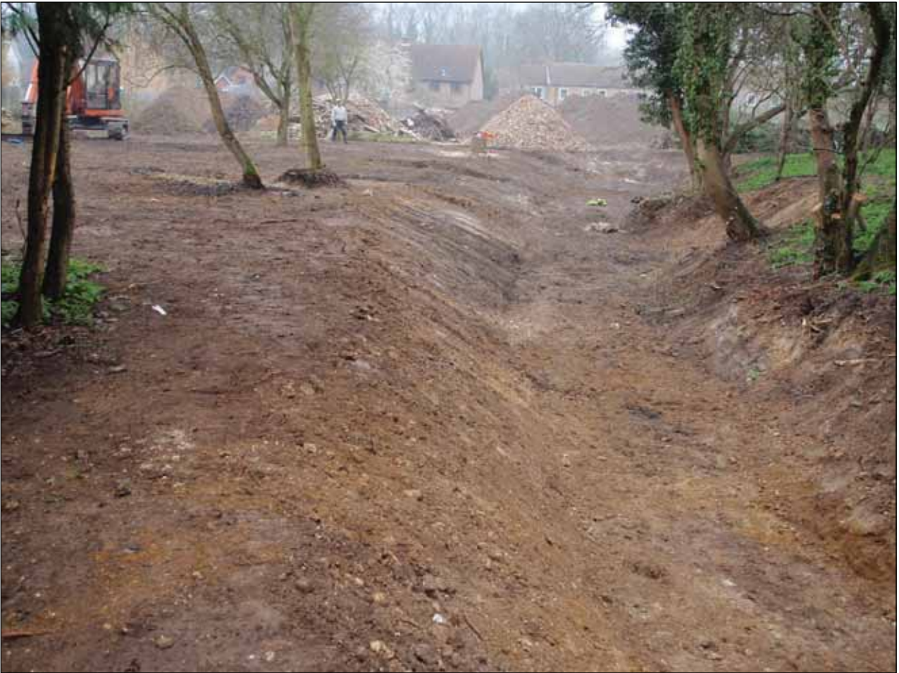
Plate 5: Western arm after works, viewed from south
