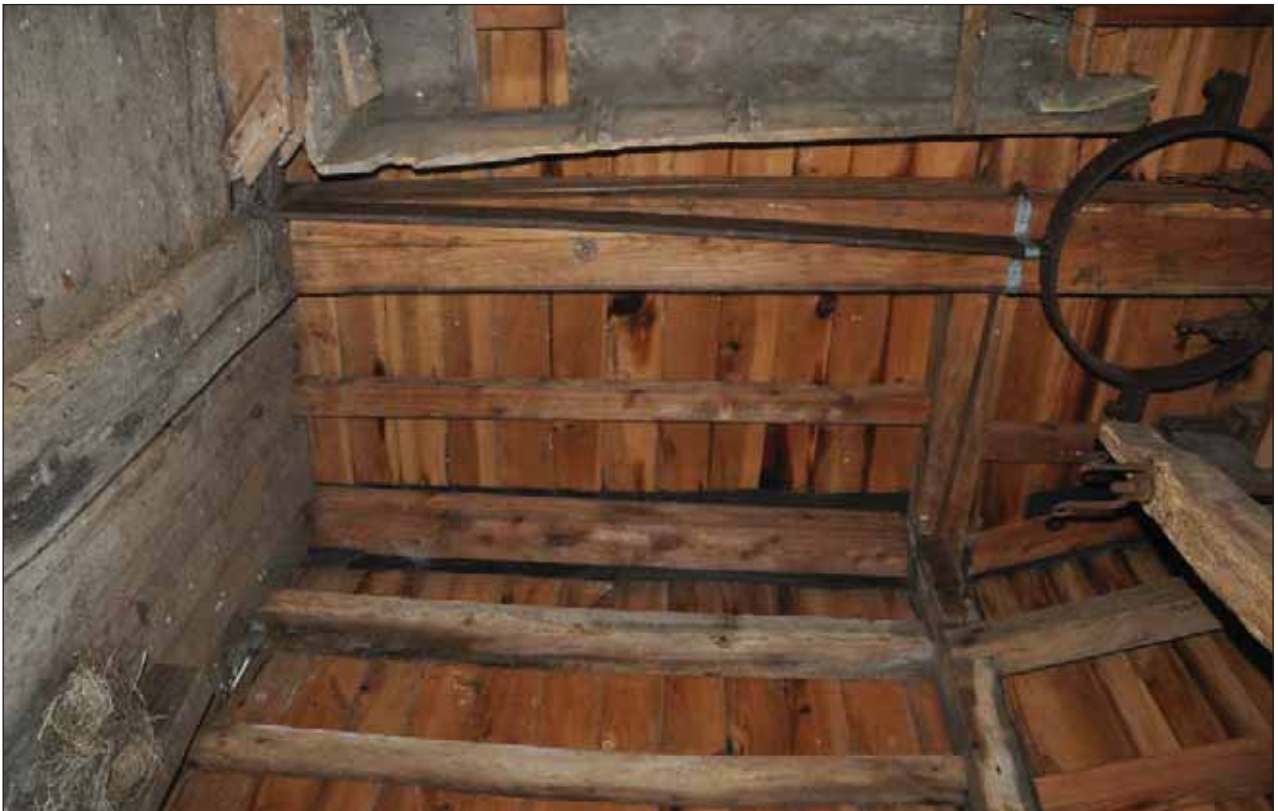
Plate 8: Large circular iron band that went around the Main post.
