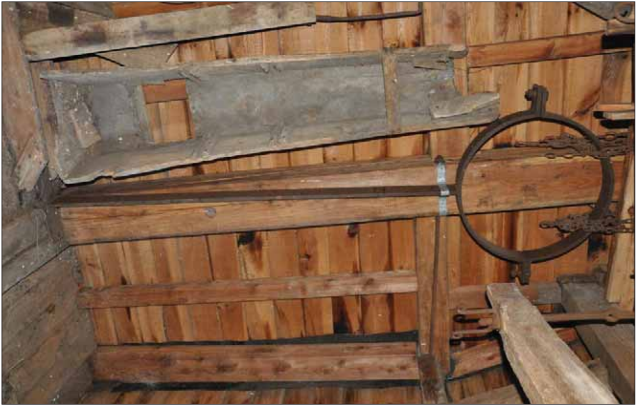
Plate 13: Large circular iron band that went around the Main post.spout.
