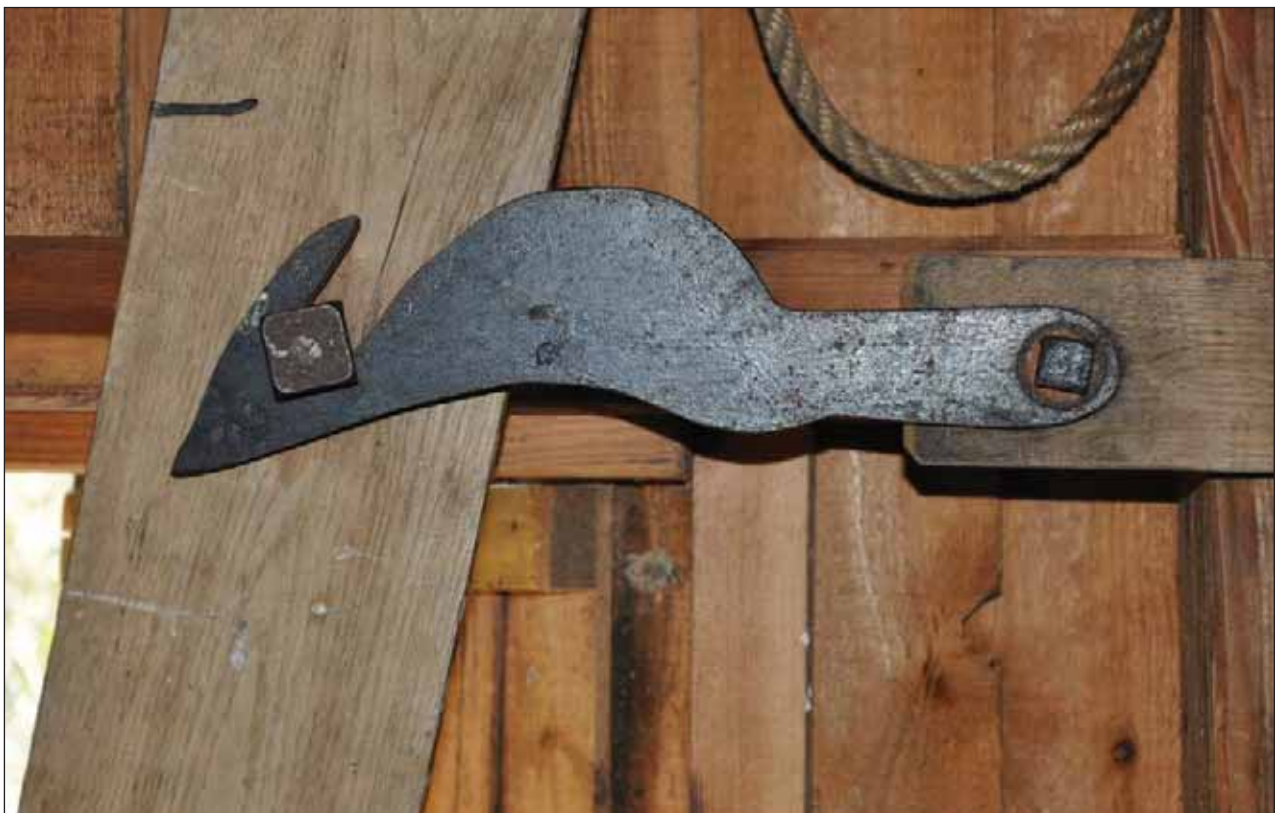
Plate 50: Metal hook to hold brake-lever in "brake not engaged" position.
