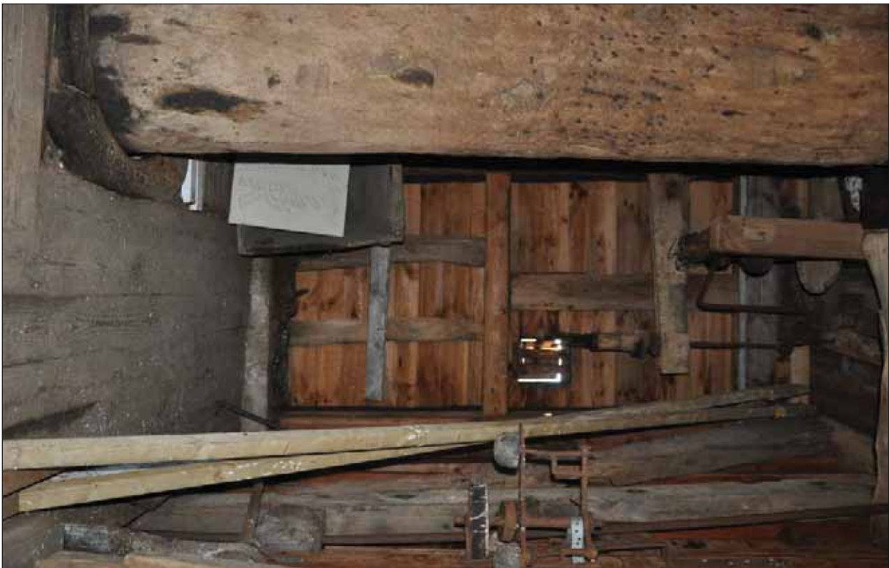
Plate 9 Meal floor looking forward. Showing Lag Governor attached to the wall. wooden grain spout.
