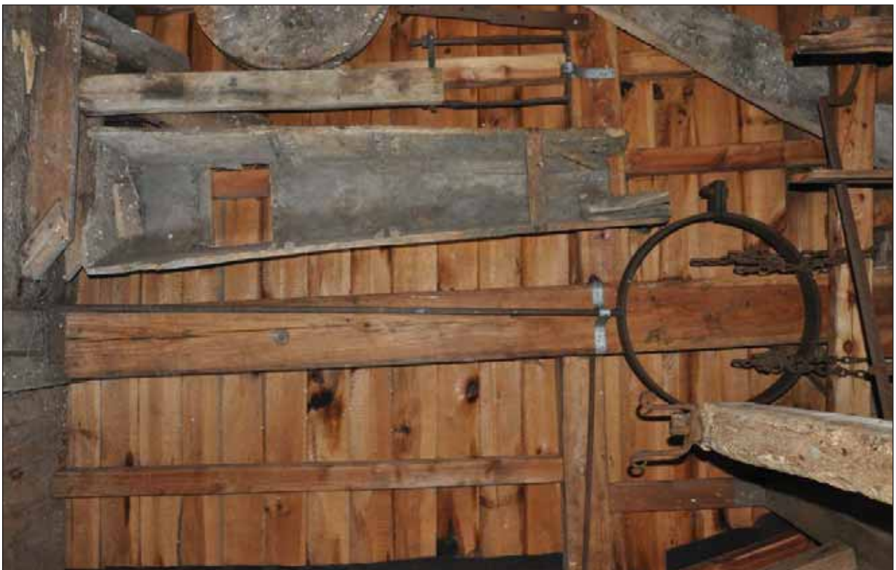
Plate 14: Large circular iron band that went around the Main post with long bar attached.
