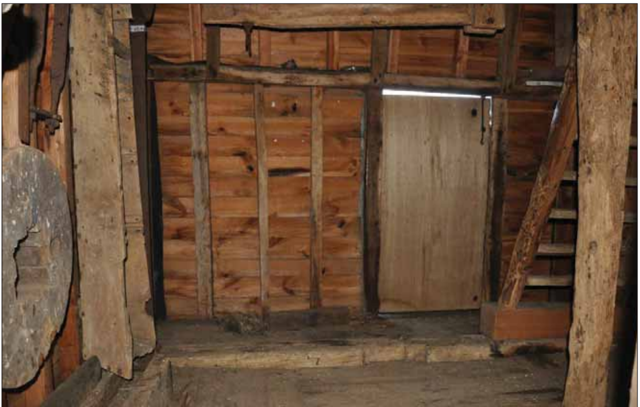
Plate 66: Rear wall and door leading to outside step ladder. Door closed. side of roof at front
