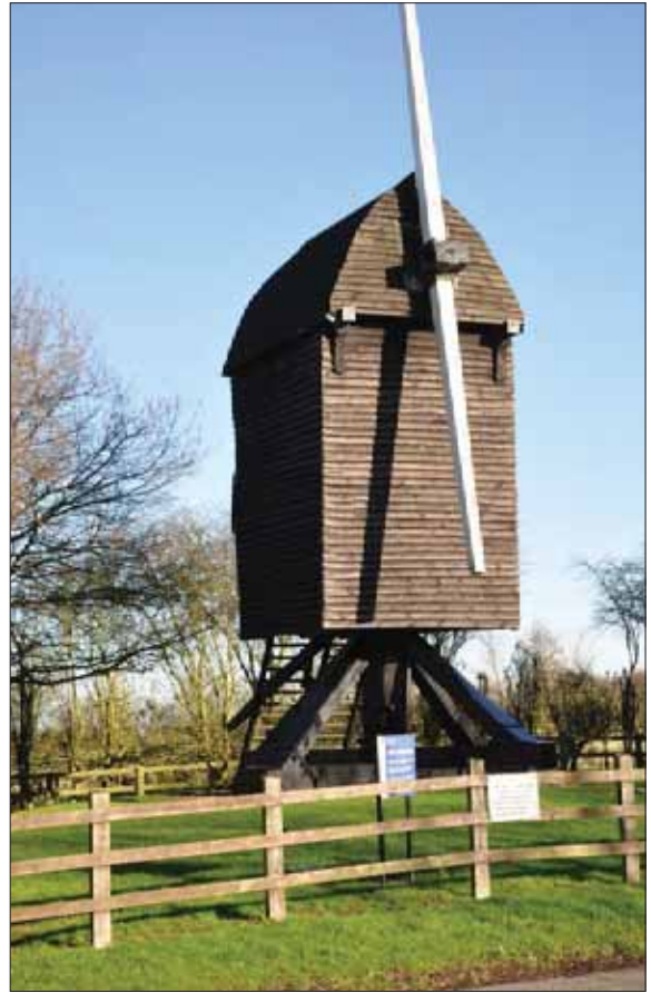
Plate 5: Buck and Trestle, one Stock in place front of mill.
