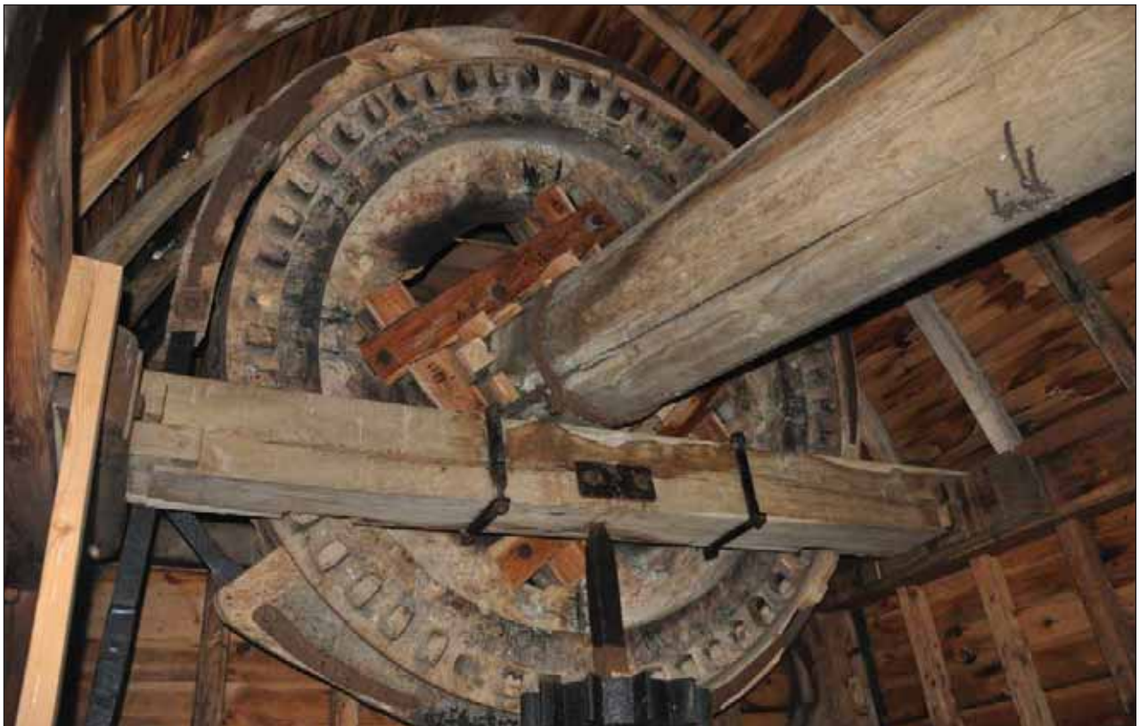
Plate 42: Brakewheel , windshaft and Sprattlebeam.
