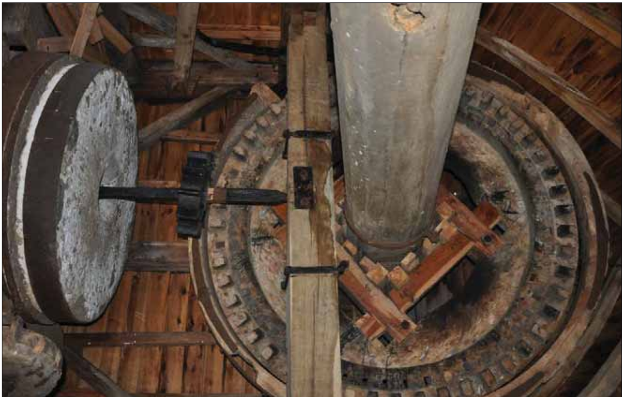
Plate 54: Brakewheel, windshaft and Sprattlebeam. Stone nut not engaged.
