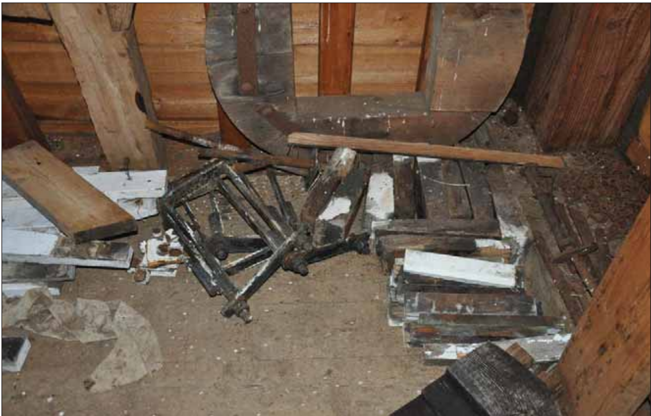
Plate 28: Sail clamps from the 1981 sails; also wooden wedges.
