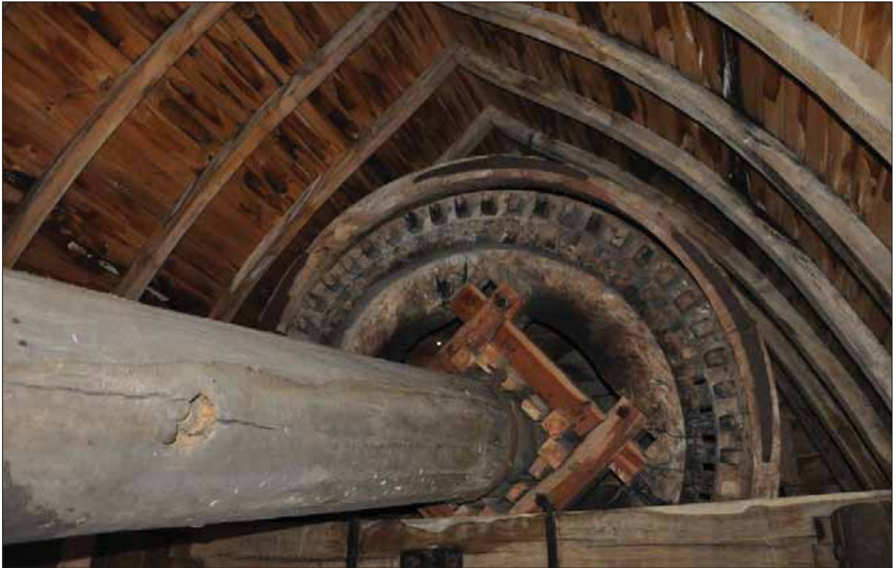
Plate 55: Brakewheel , windshaft and upper surface of Sprattlebeam
