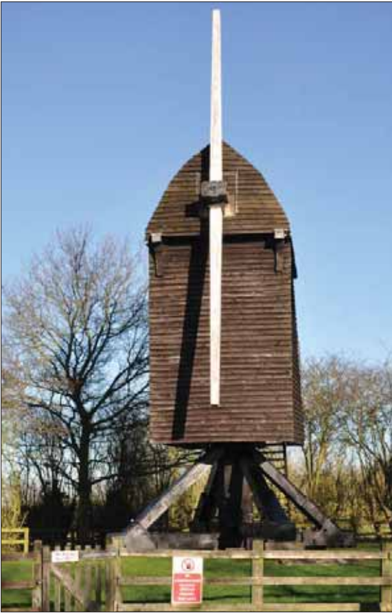
Plate 4: Buck and Trestle, one Stock in place front of mill.
