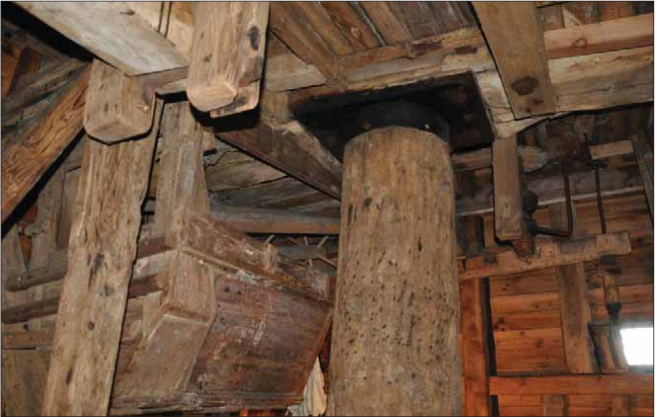
Plate 63: Samson Head and Upper part of Main Post
