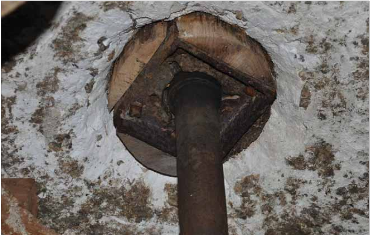
Plate 25: Stone spindle under front set of stones.
