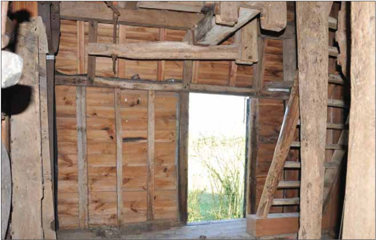
Plate 65: Rear wall and door leading to outside step ladder. Door open.
