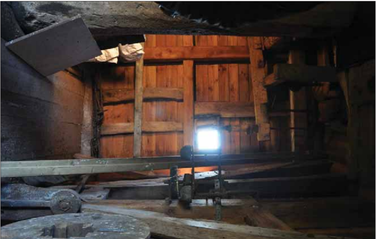
Plate 62: Meal Floor- right-hand side looking forwards showing open hatchside of roof at front
