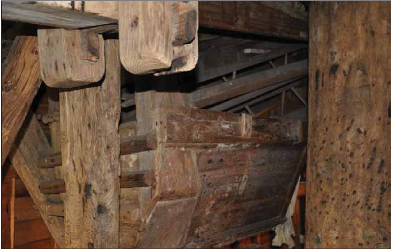
Plate 35: Flour bolter - oblique rear view.
