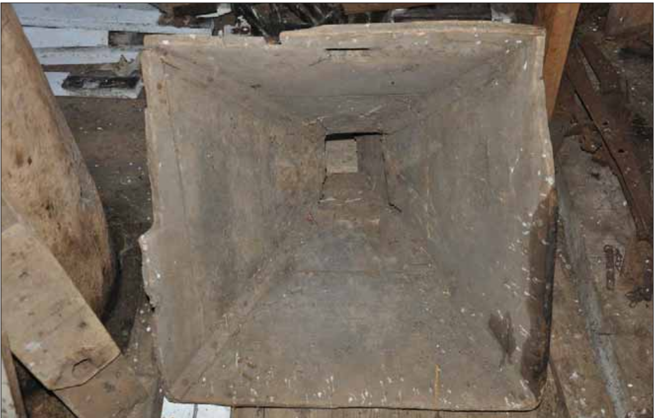
Plate 32: Hopper to feed grain into centre of top of a millstone.
