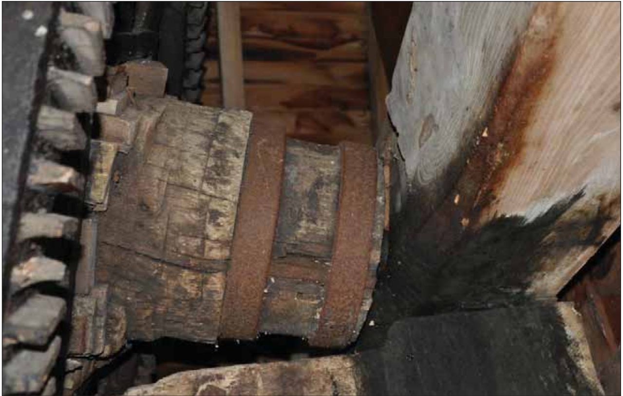
Plate 53: Rear end of Windshaft and rear face of Tailwheel.
