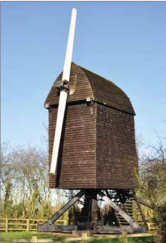
Plate 6: Buck and Trestle, one Stock in place front of mill. South east
