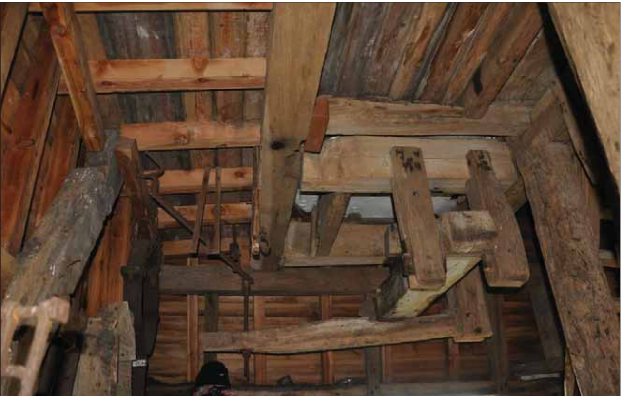
Plate 64: Rear Stones from below, including Bridge Beam and tentering Gear supports
