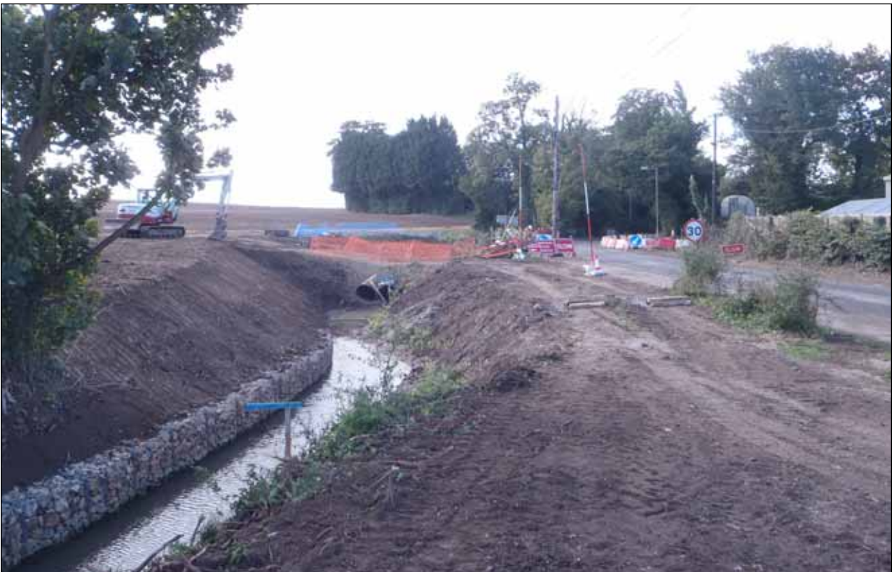
Plate 8: Helions Brook widening excavations
