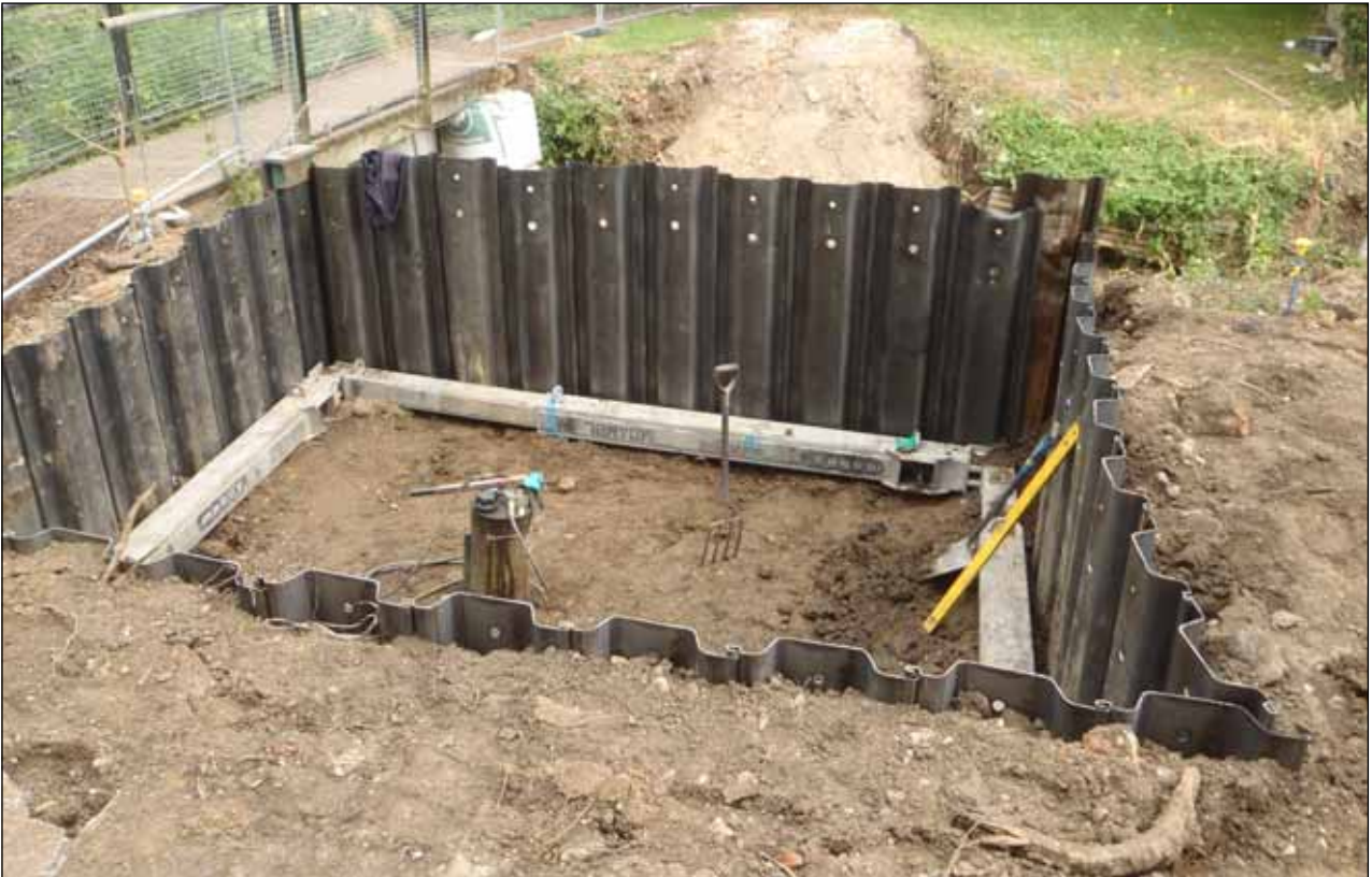
Plate 5: Excavations at the private access footbridge
