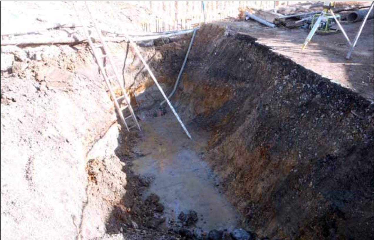
Plate 7: Water Lane culvert excavations
