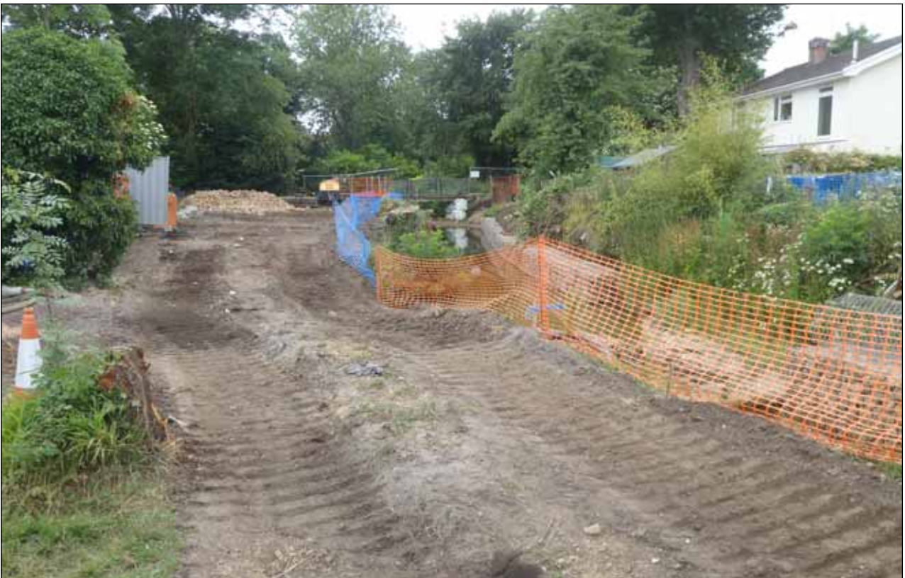
Plate 6: Churchfield footbridge excavations
