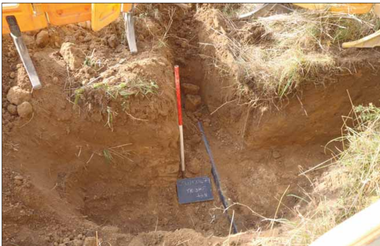
Plate 1: Excavations for watermain extension, facing west
