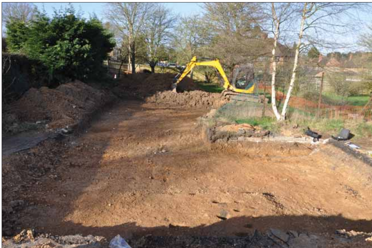
Plate 17: Excavation are being machine stripped
