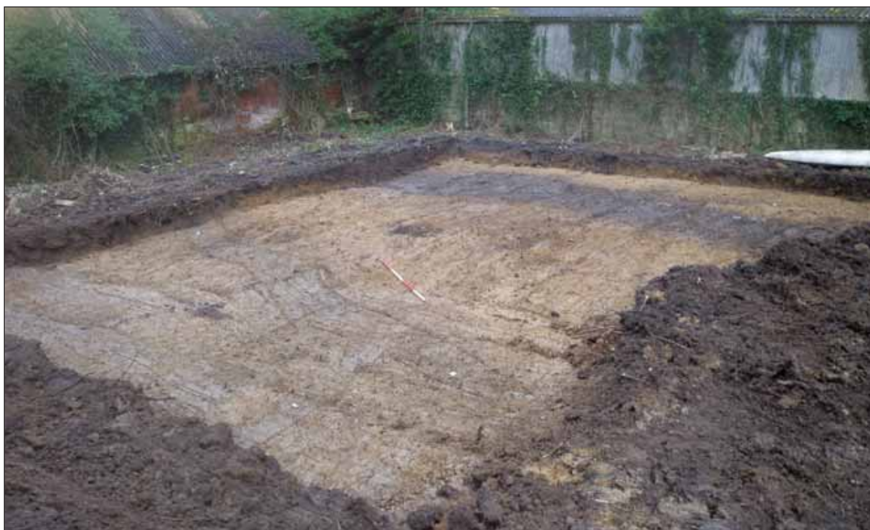
Plate 1: Pre-excavation shot of west side of site, from the north-east
