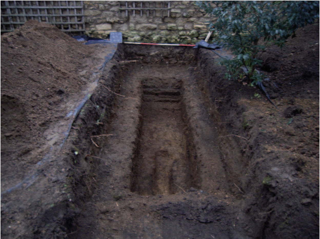
Plate 3: General view looking S of excavated features in Trench 3
