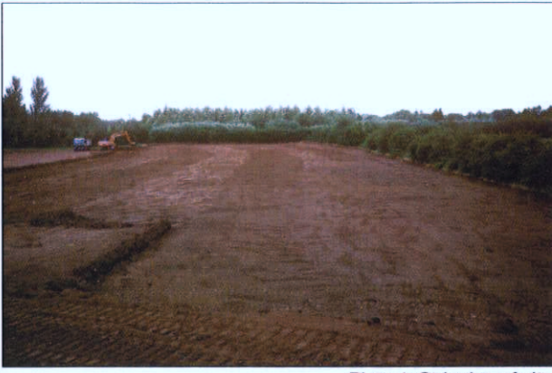
Plate 1: Stripping of site
