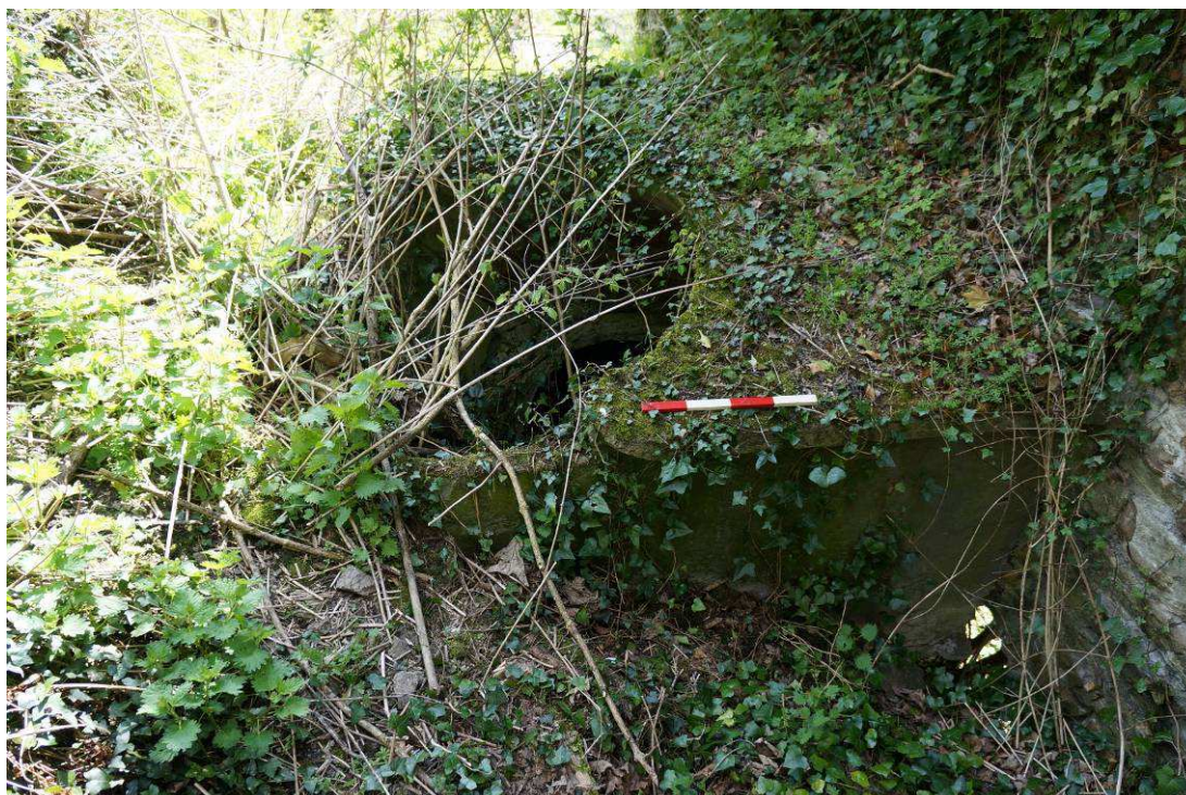
Plate 20: The circular opening leading into the side flue (Site 51b)
