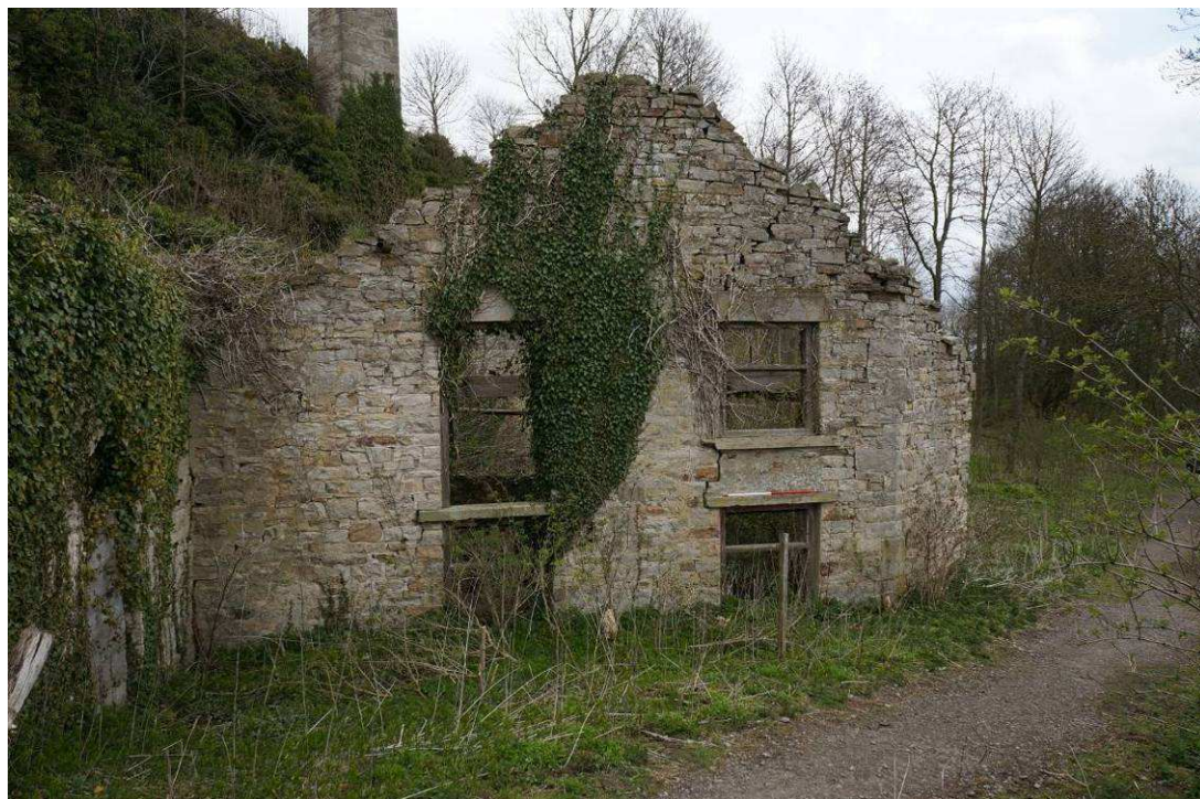
Plate 22: The western elevation of the Boiler House (Site 53)
