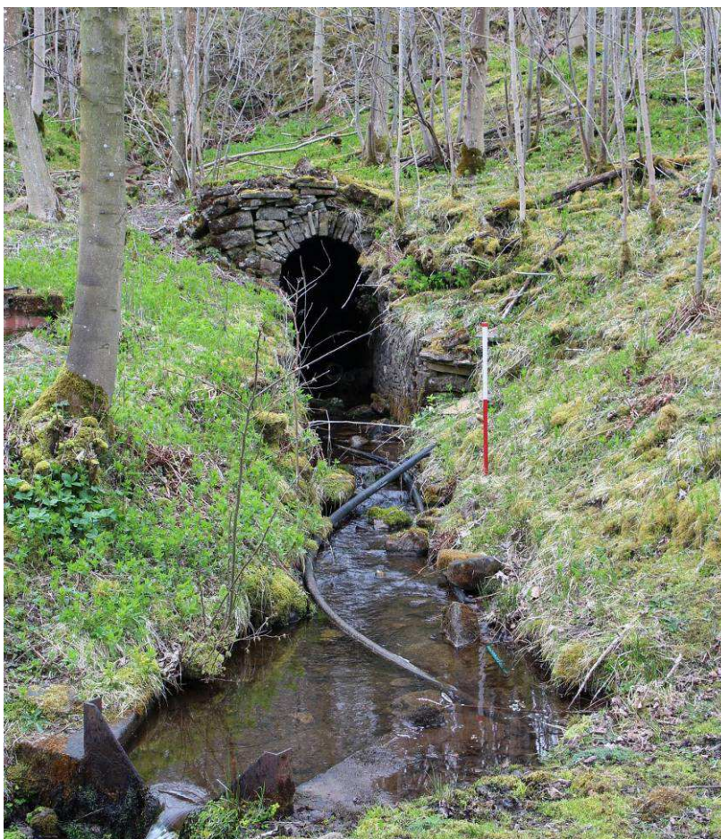
Plate 10: Adit entrance - Site 16
