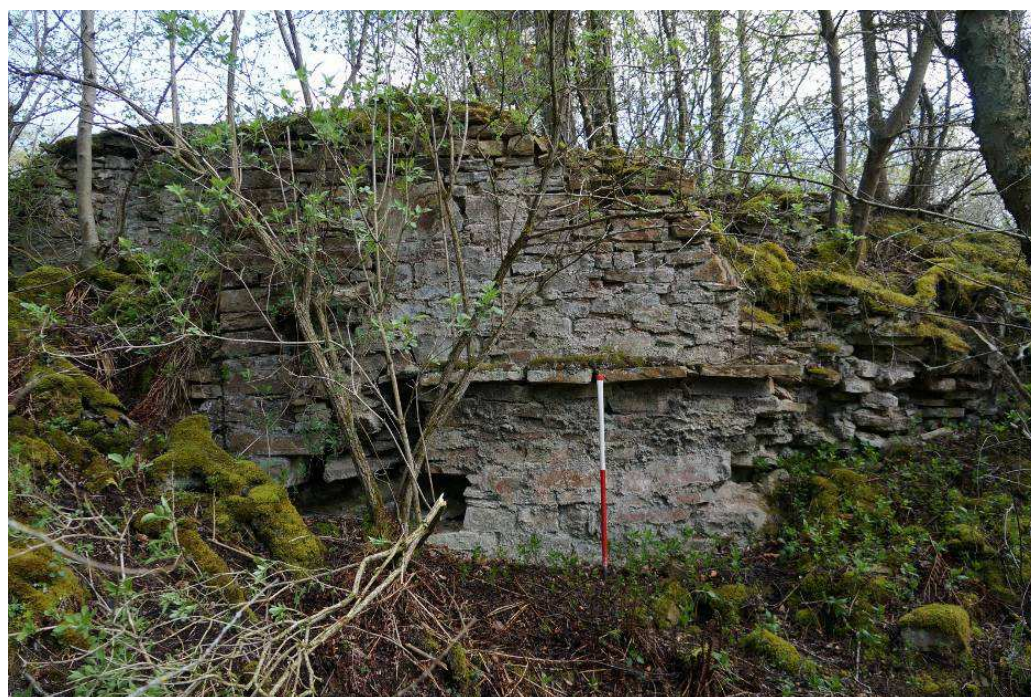
Plate 48: The western face of the Condenser House (Site 102a ), where the Stokoe Condenser formerly butted (Site 102d )
