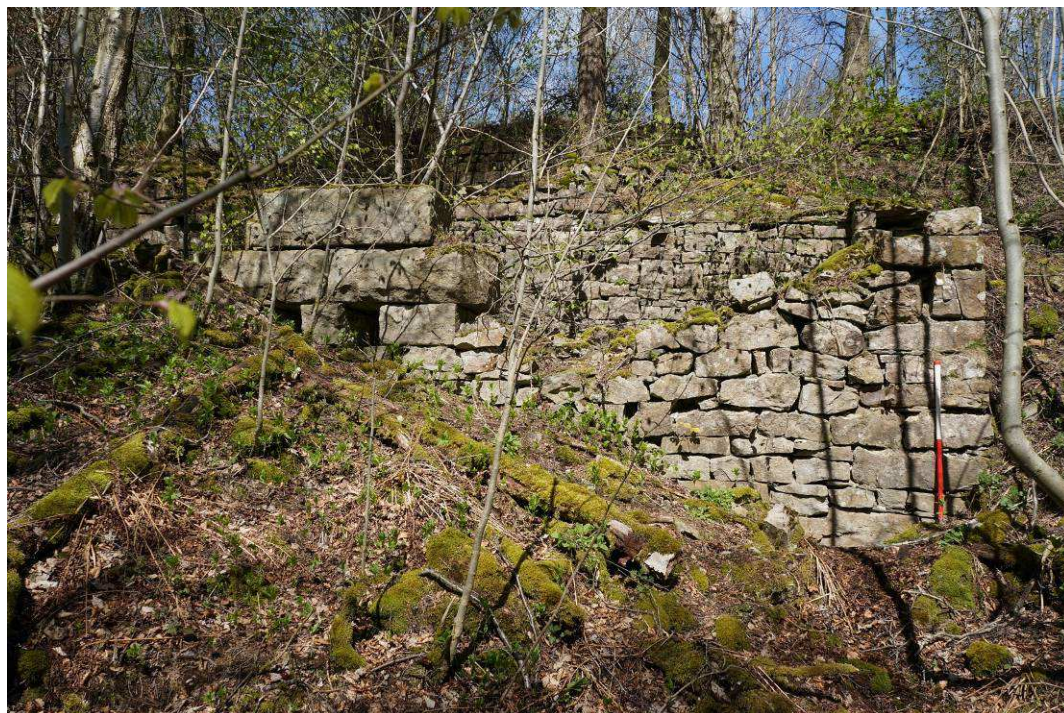
Plate 46: The southern side of the Condenser House wheel-pit (Site 102a)
