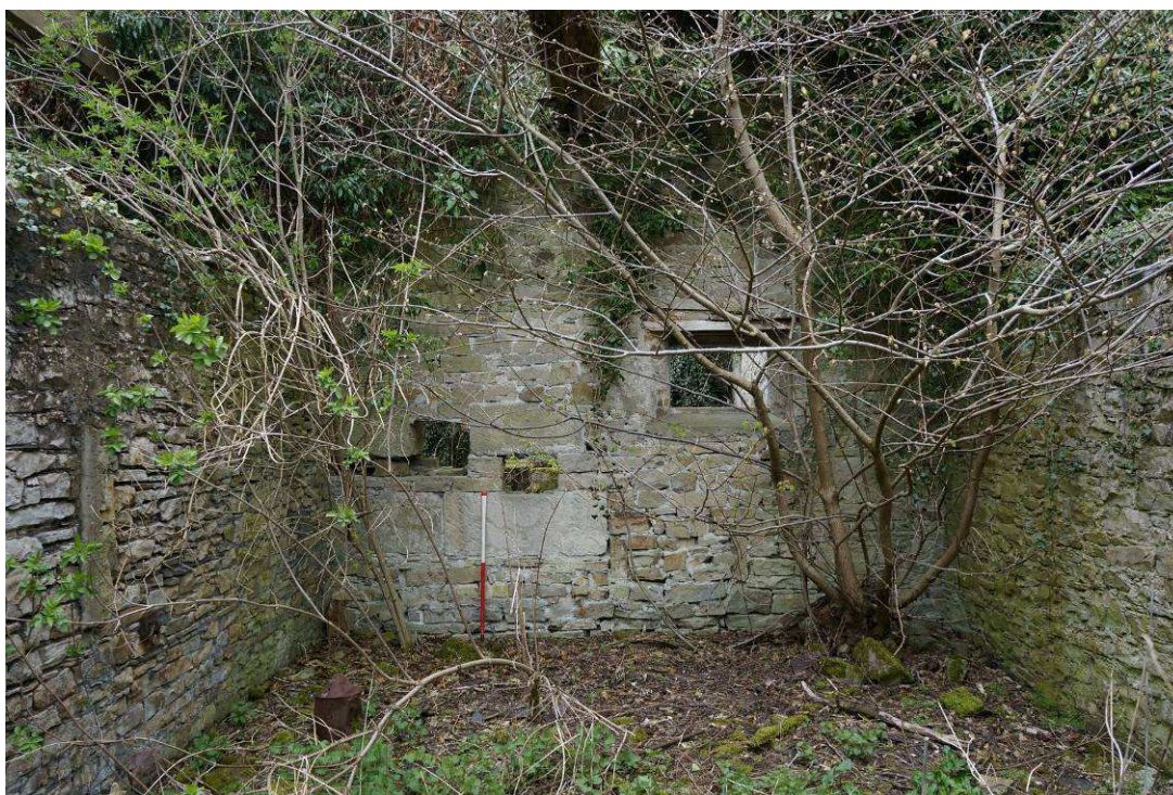
Plate 21: The interior of the central cell of the Boiler House (Site 53 ), looking north
