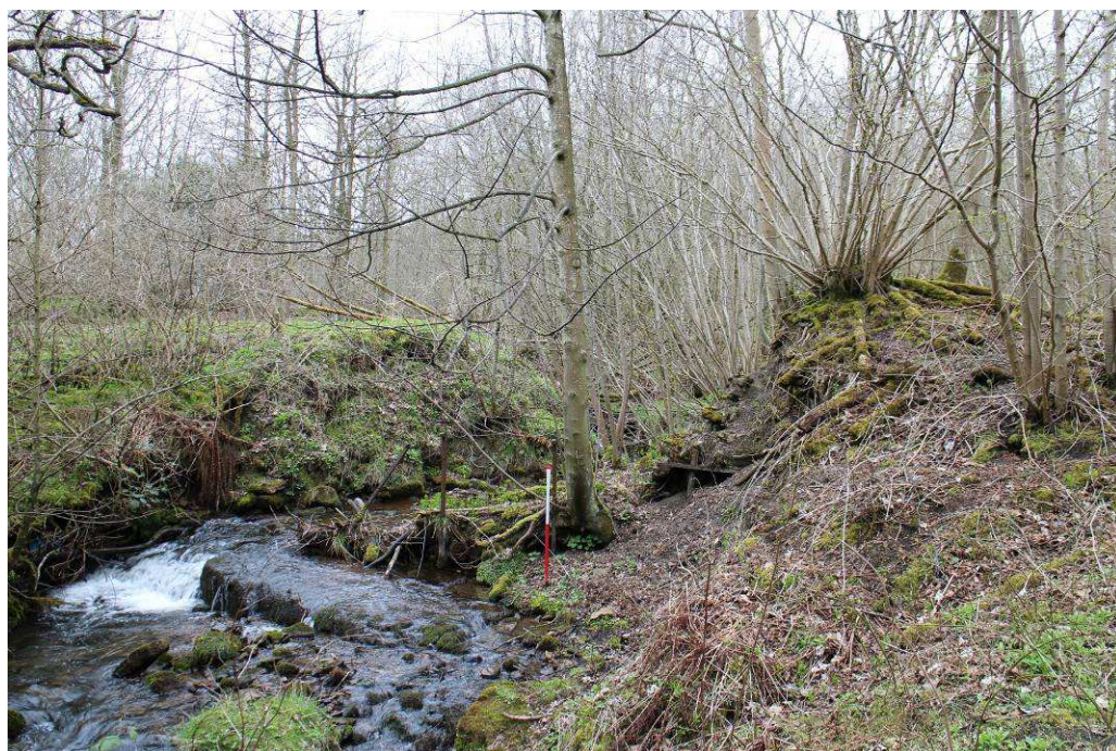
Plate 52: The extant section of the dam (Site 90 ) which has been breached
