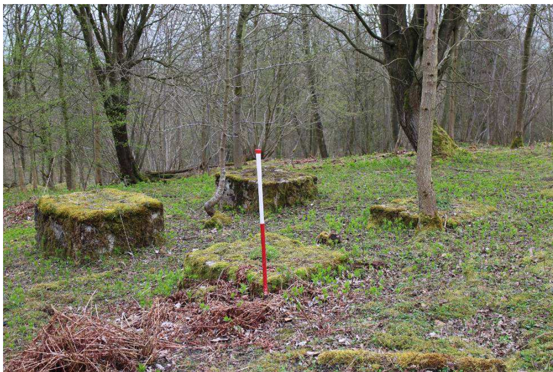
Plate 55: Concrete Aerial Ropeway Base (Site 4 )
