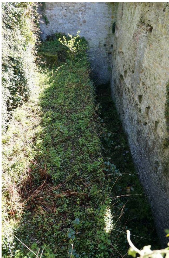
Plate 18: Interior of the Engine House (Site 66 ), looking east
