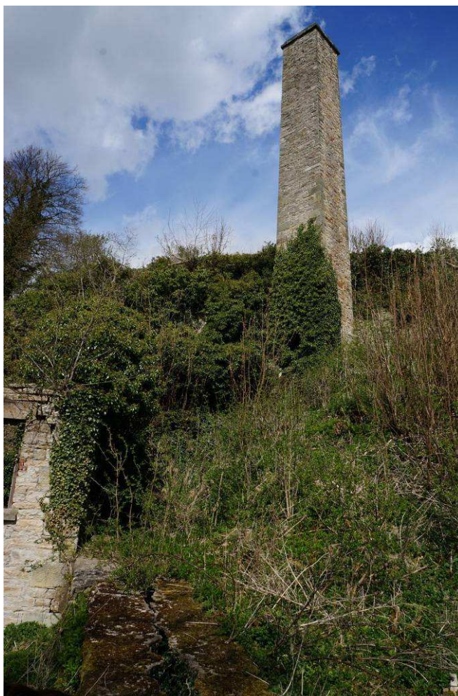
Plate 24: The chimney (Site 52 ) and flue (Site 51a ) looking north
