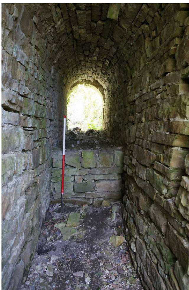
Plate17: The barrel-vaulted tunnel (Site 67) for drive shafts/connecting rods between the Engine House and mine shaft.
