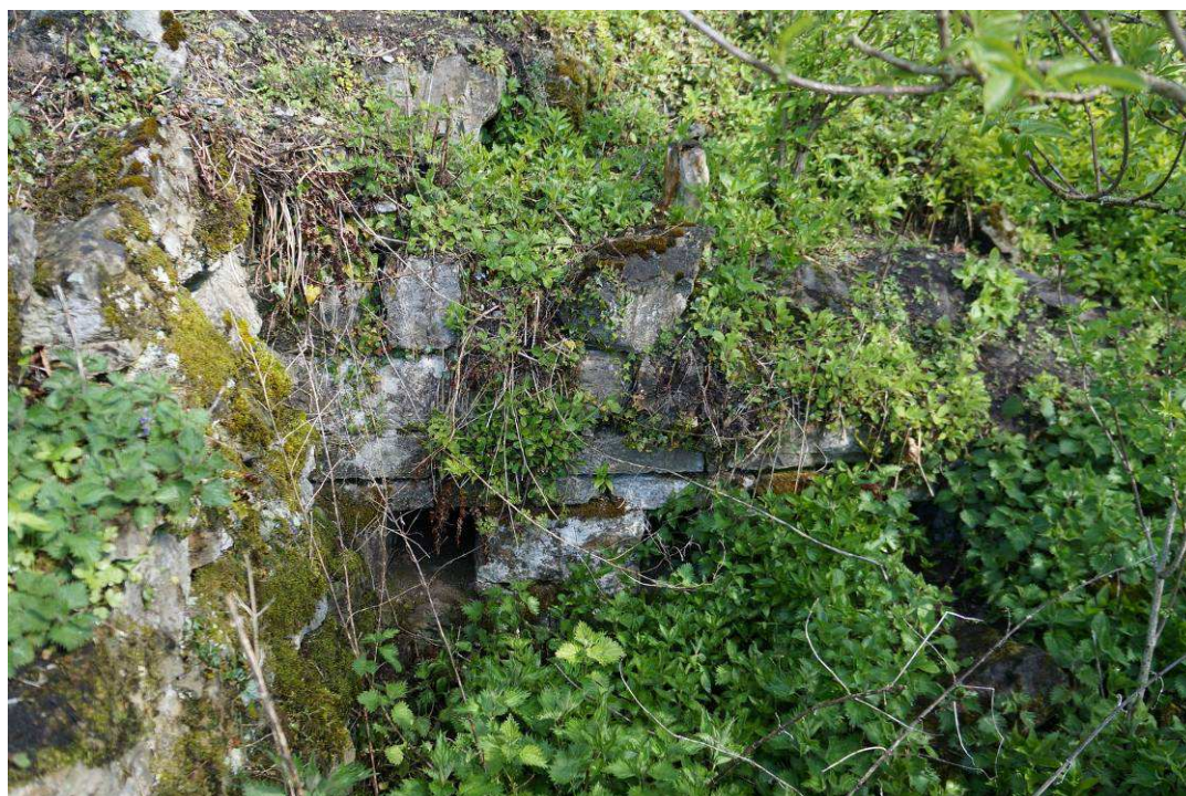
Plates 16: One of a series of square slots set into the walling at the east end of the wheel-pit (Site 65 )
