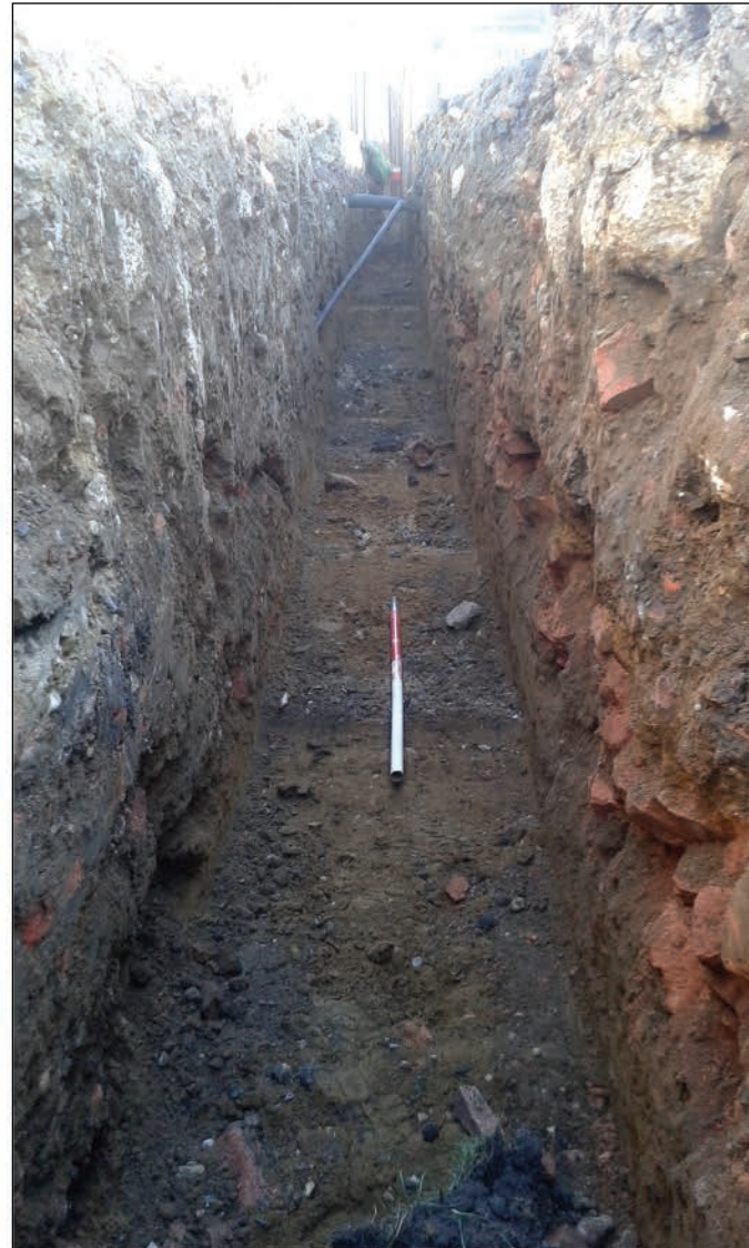
Plate 7: Trench run looking west
