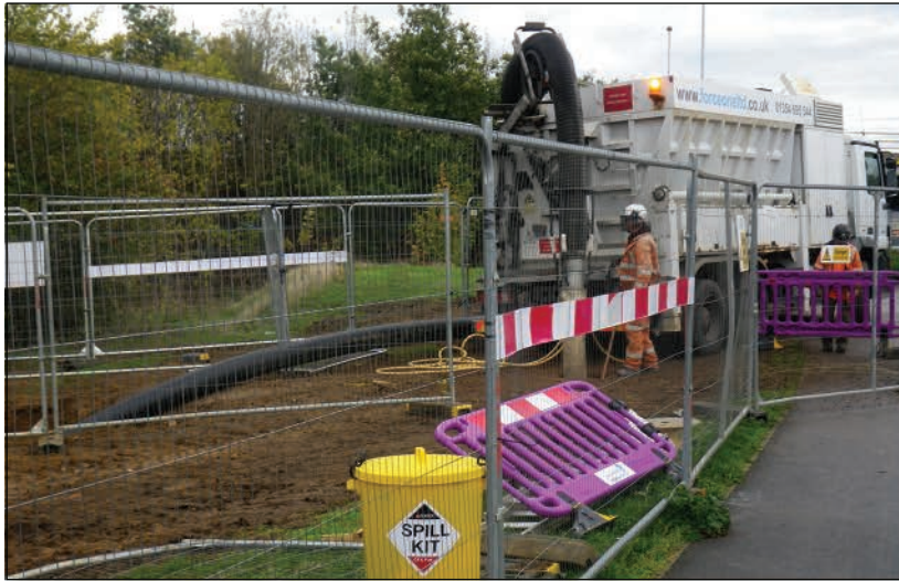
Plate 1: Test Pit 1 Suction excavation
