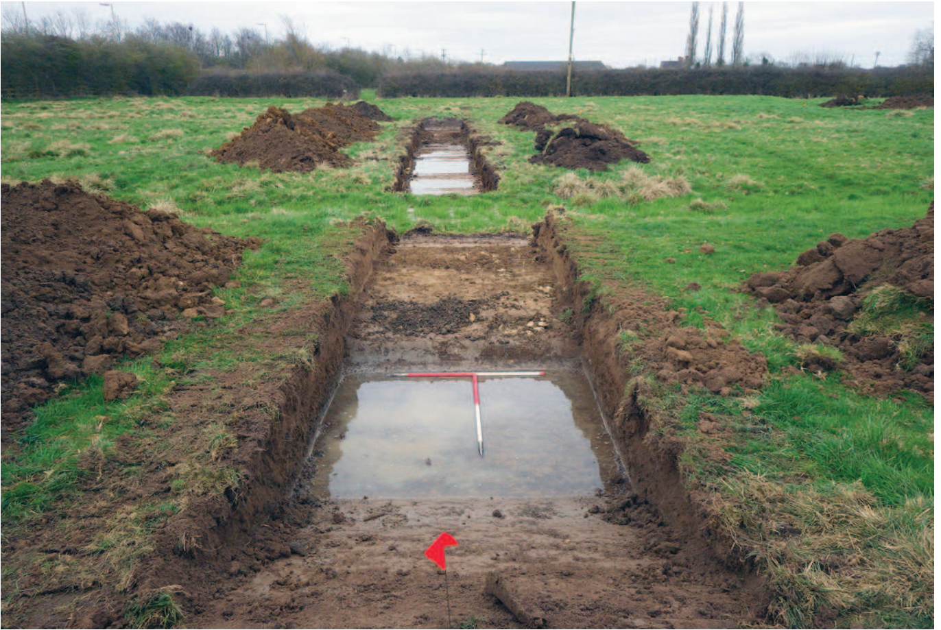
Plate 3: Trench 2 view north-east along the trench
