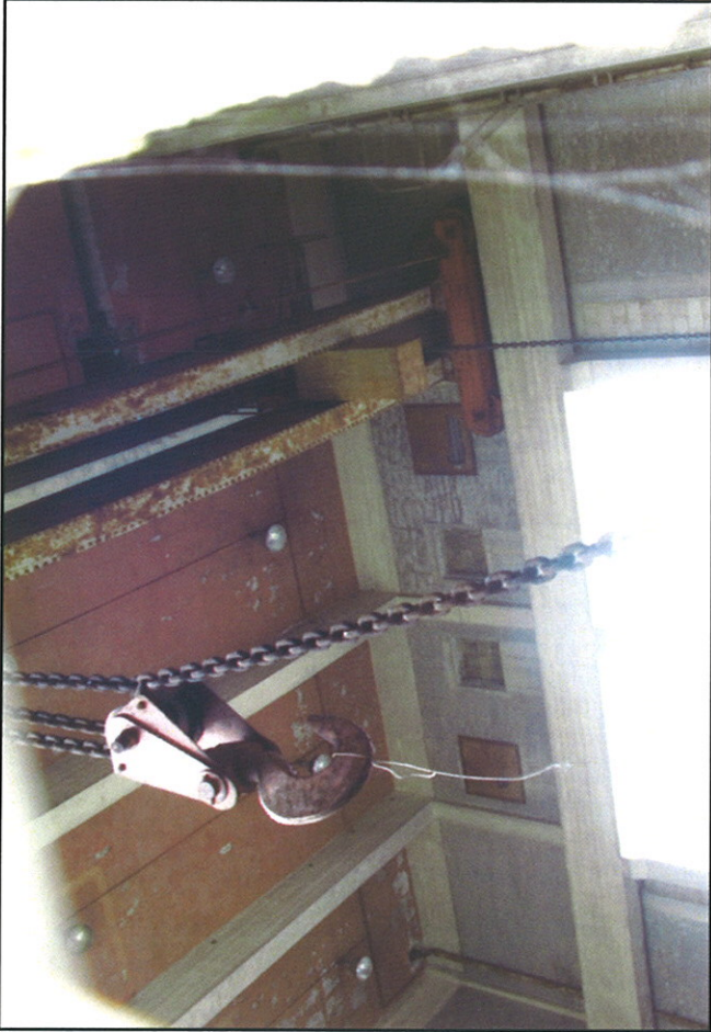
Plate 13: No. 2 (Koepe) Winder House, interior looking east
