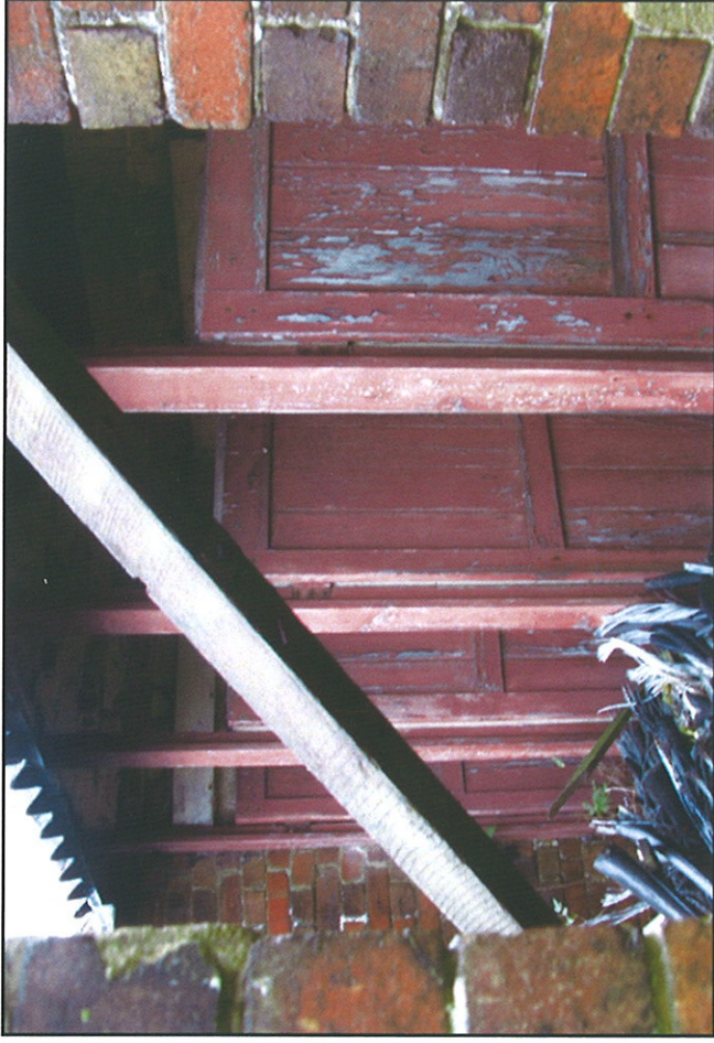
Plate 34: Building 12, lavatory cubicle doors
