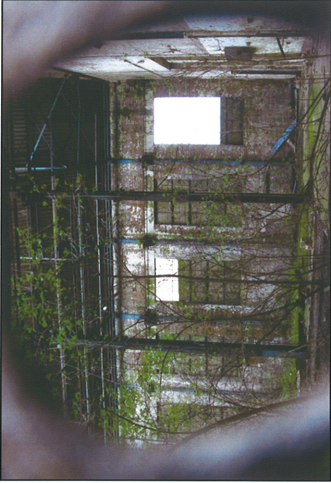
Plate 46: Building 19, interior looking south-east
