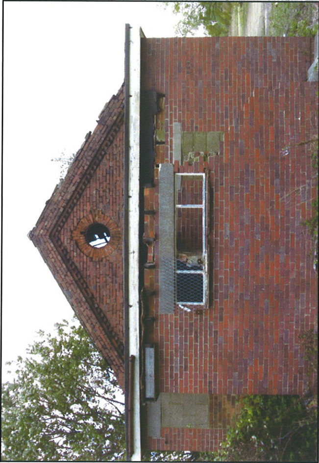
Plate 25: Building 9, south-west gable and later extension
