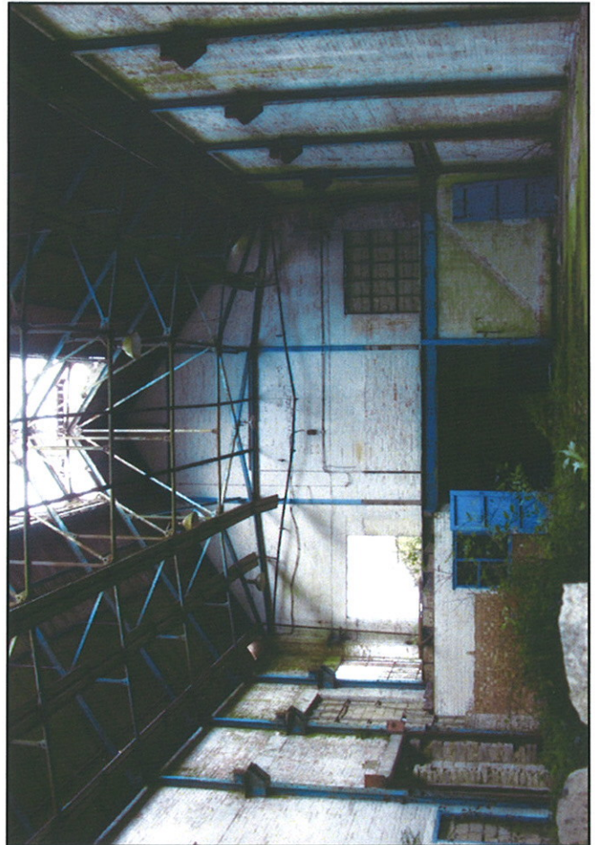
Plate 43: Building 17, interior looking north-west
