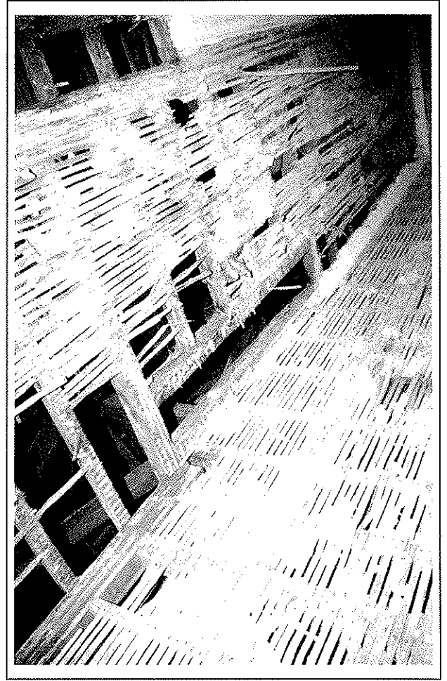
Plate 25: Trimming within ceiling above F20 suggesting former chimney
