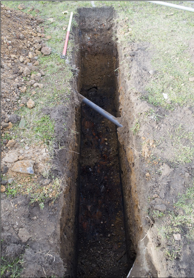
Plate 1: PT 1 looking south-east
