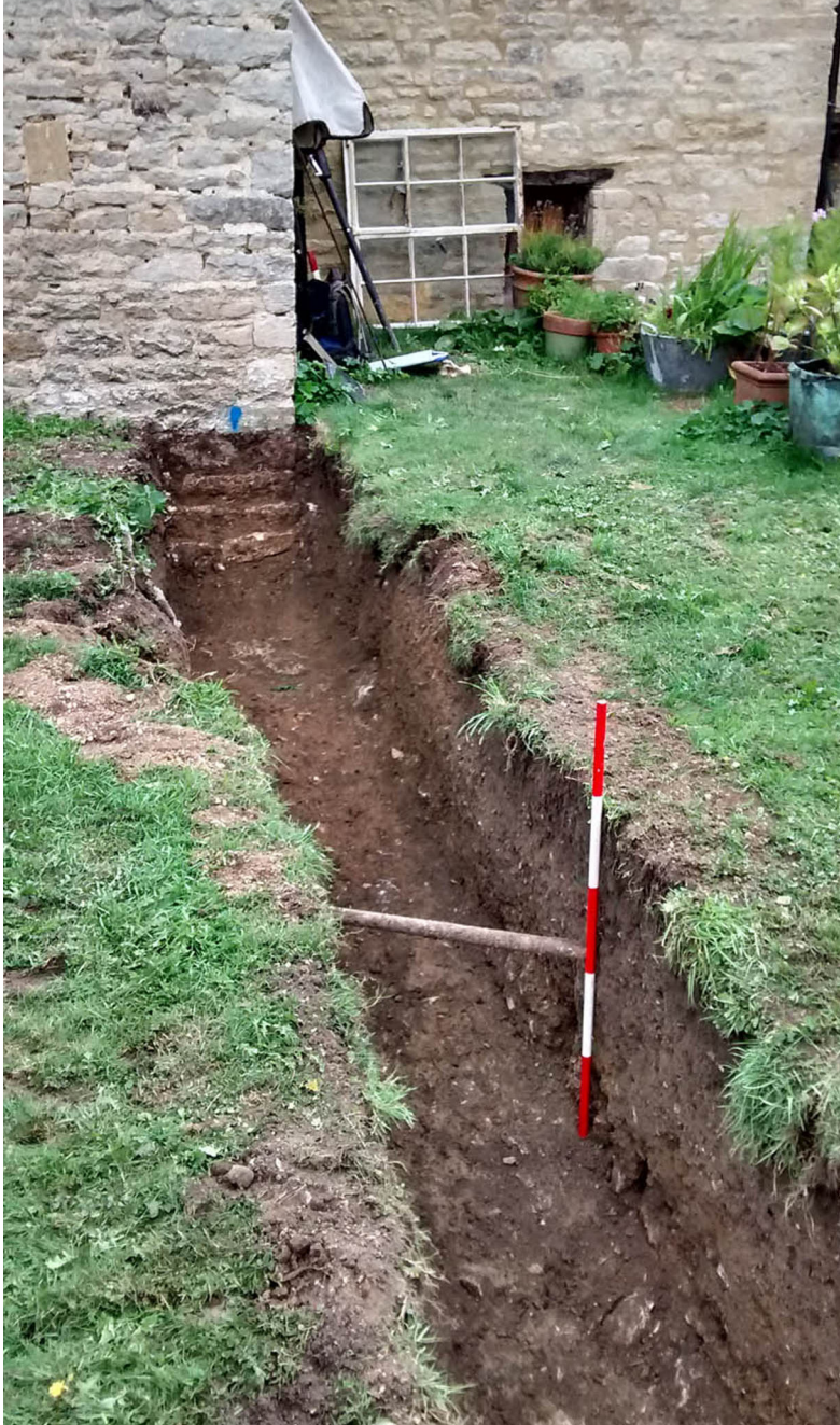
Plate 1: Foundation trench, eastern end showing wall 100, looking east
