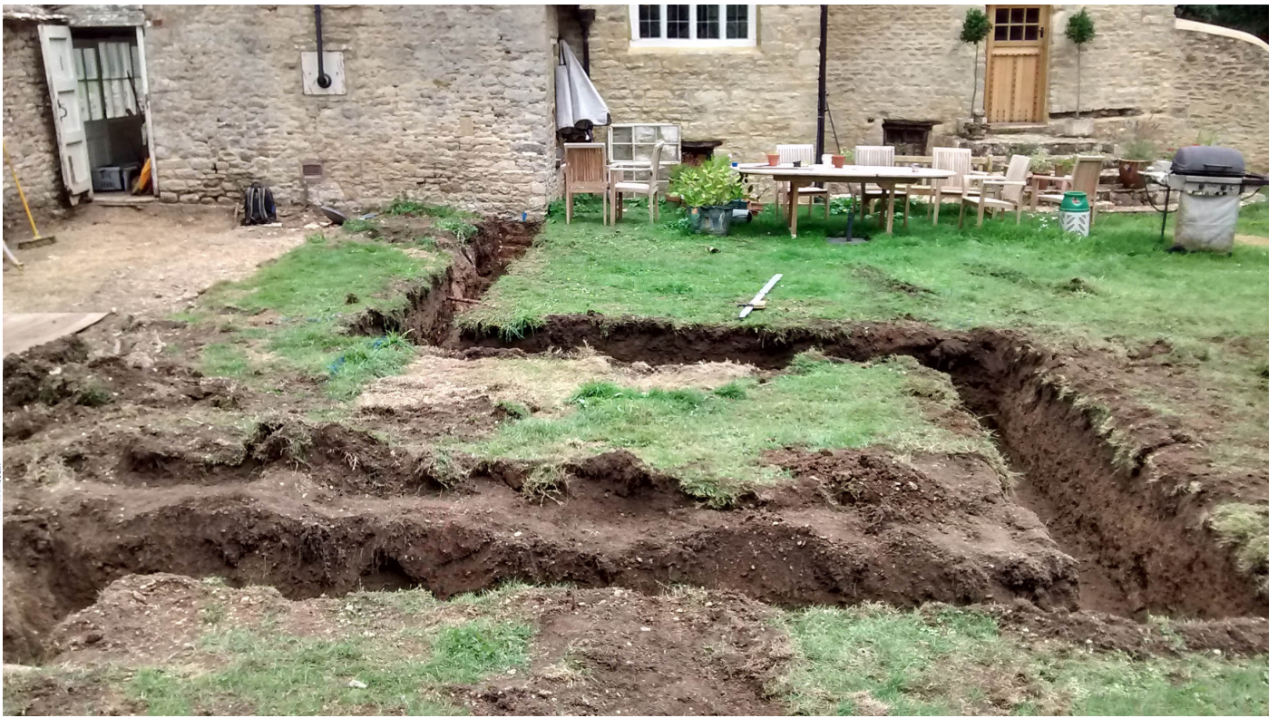
Plate 3: Foundation trenches, looking east
