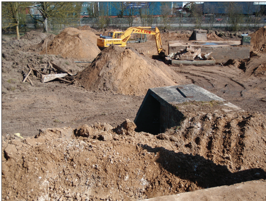
Plate 2: Concrete remains of MoD fuel depot
