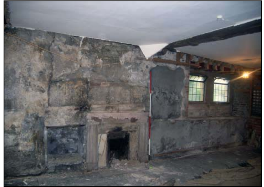
Plate 30: West elevation of Eckersley room
