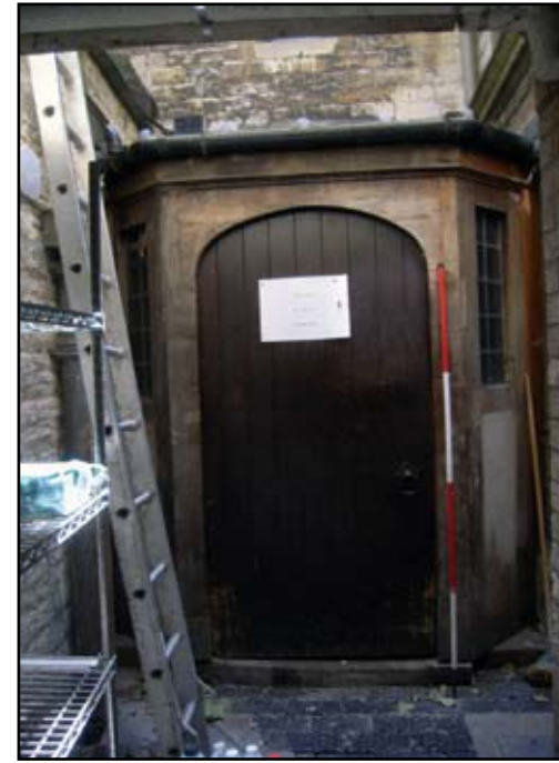
Plate 6: Entrance porch to kitchen area
