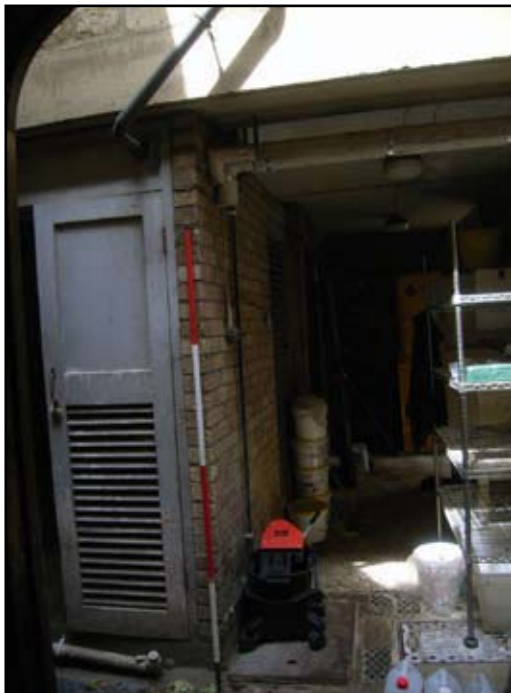
Plate 7: View of outbuildings to be demolished
