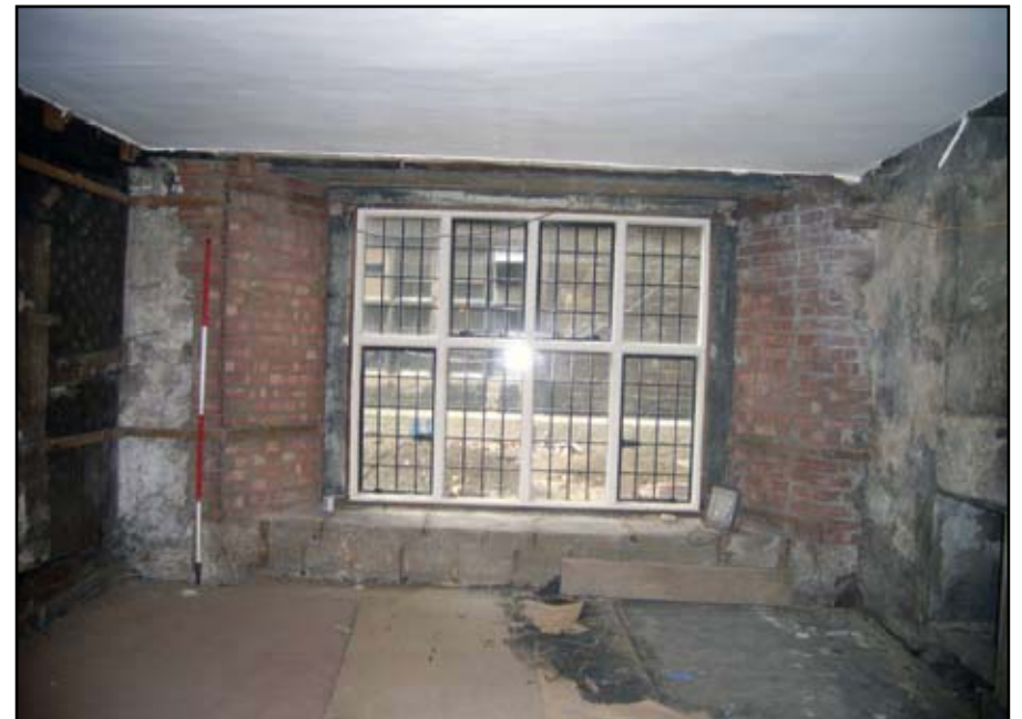
Plate 28: South elevation of Eckersley room
