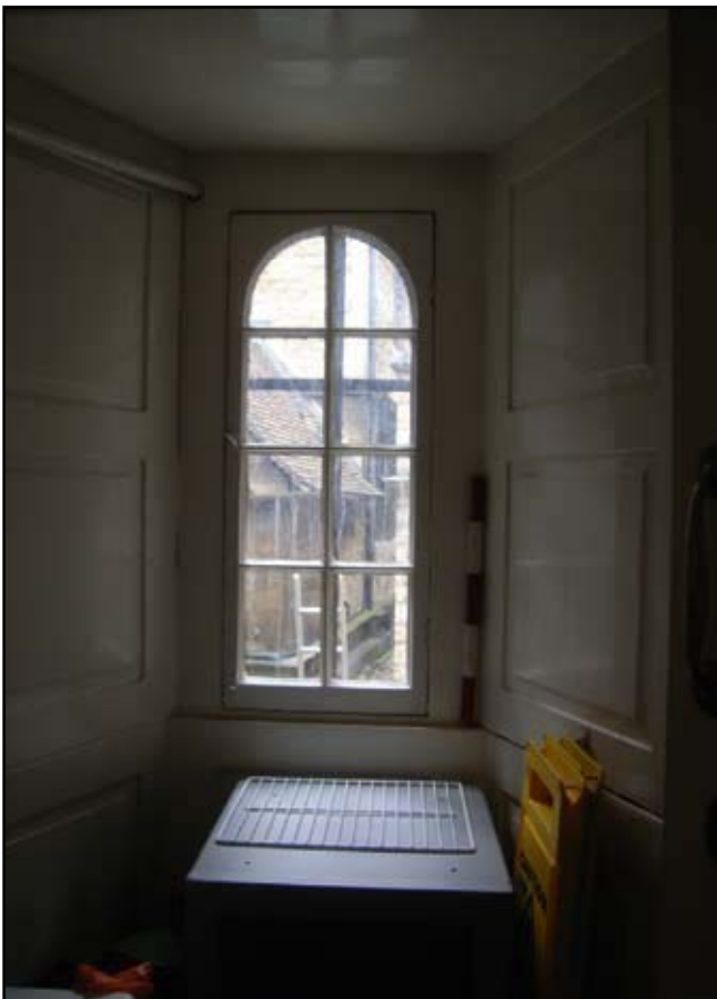
Plate 11: Detail of first floor window
