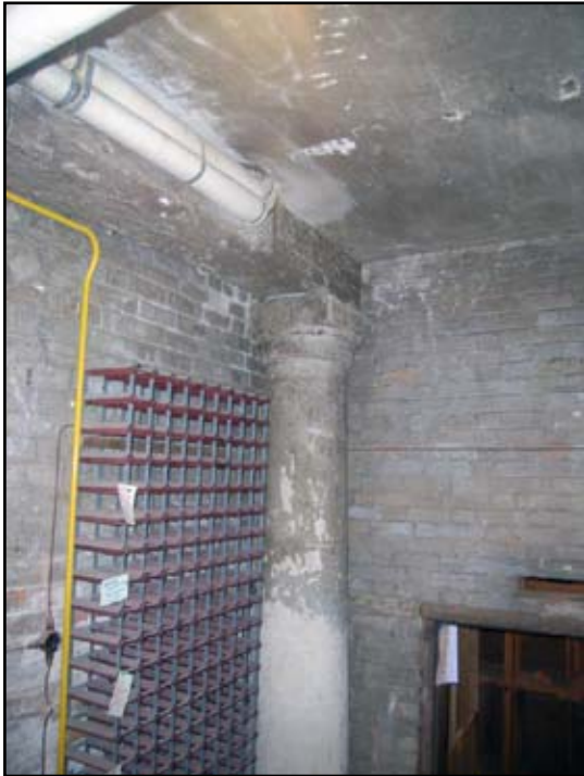
Plate 25: Detail of stone column within main Wine Cellar
