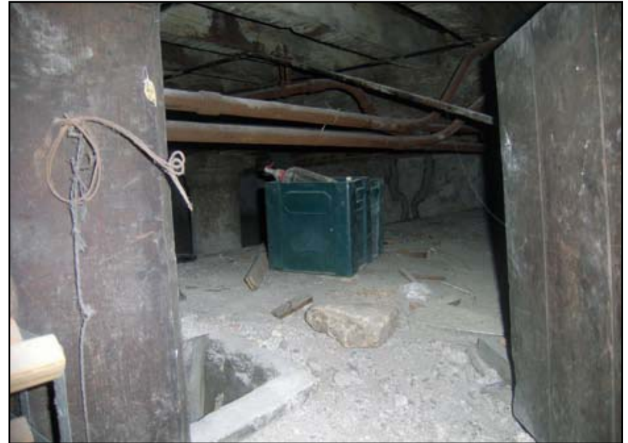
Plate 26: View of roofspace above main Wine Cellar and below hall
