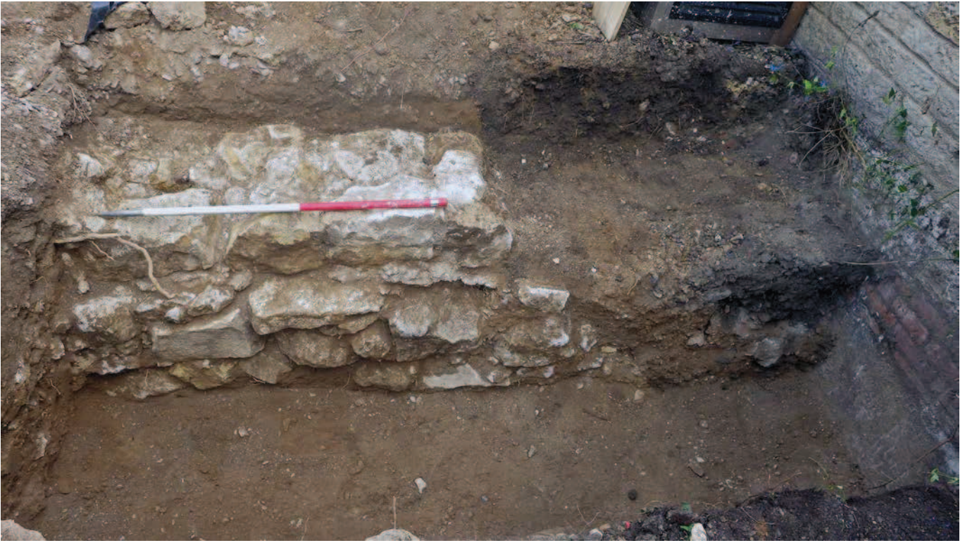
Plate 4: Wall 108 in Trench 1 prior to installation of shoring
