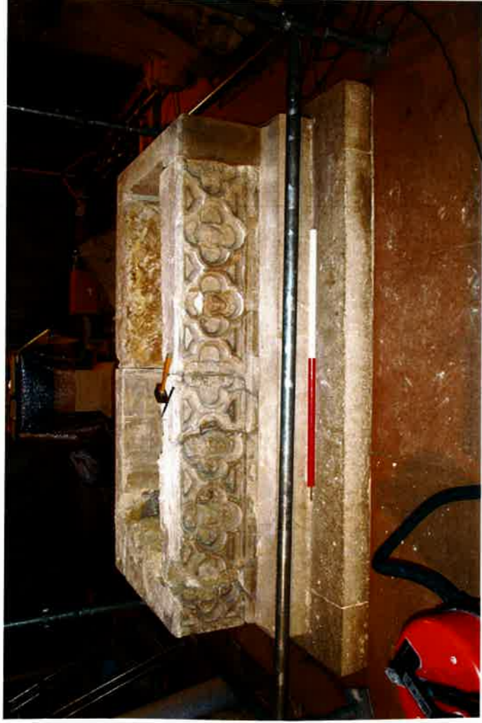
Plate 5: Exterior of shrine, showing sides, steps and replacement stonework looking North
