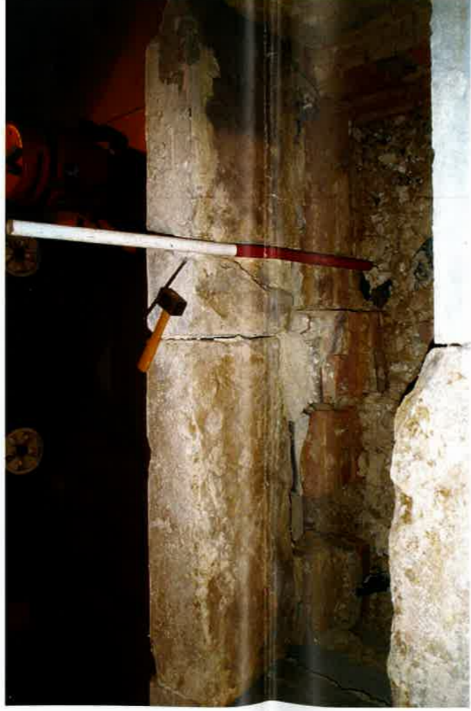
Plate 3: Internal view of shrine showing construction looking Southward
