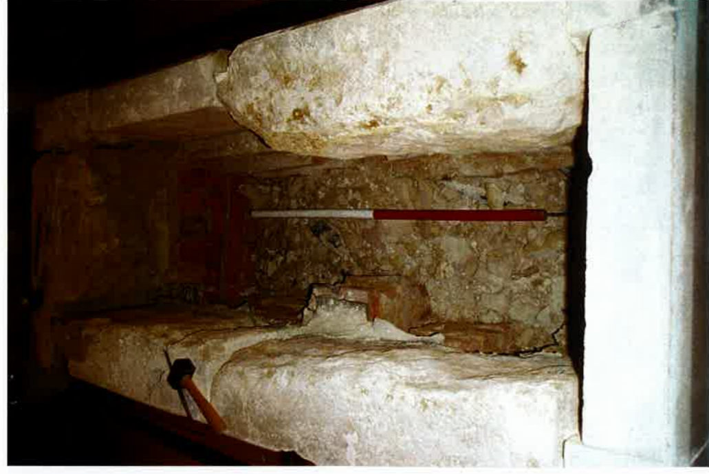
Plate 2: Internal view of shrine showing construction looking westward
