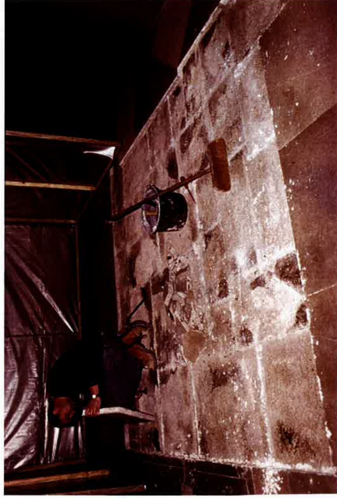
Plate 1: Slabs removed for new base for shrine
