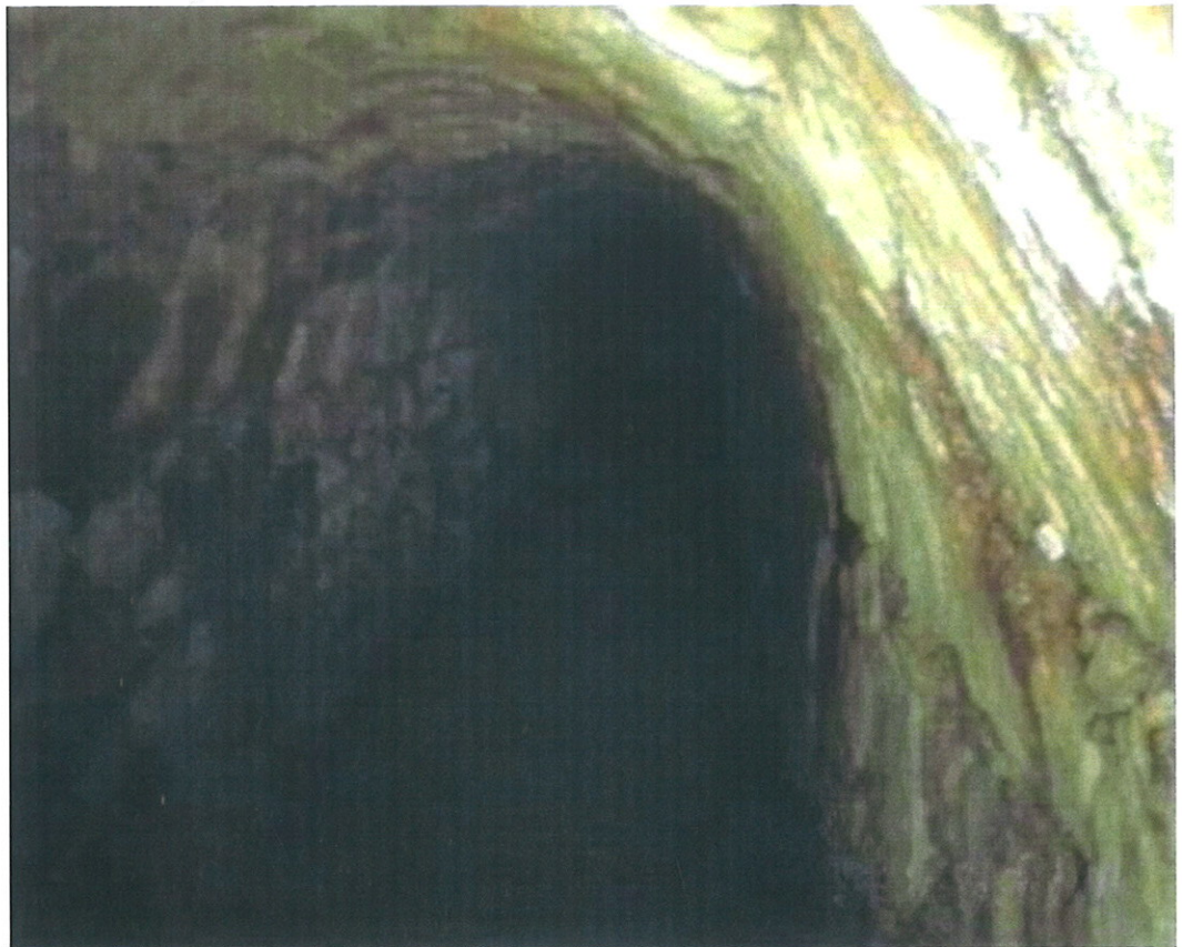
Plate 2: Interior of the culvert, facing south-east from manhole 32
