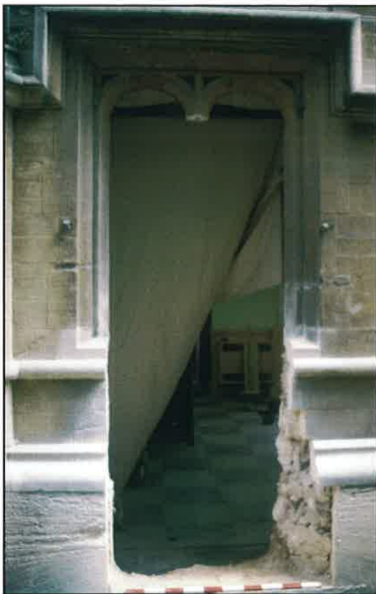
Plate 5: External view following removal of window and stonework, west elevation
