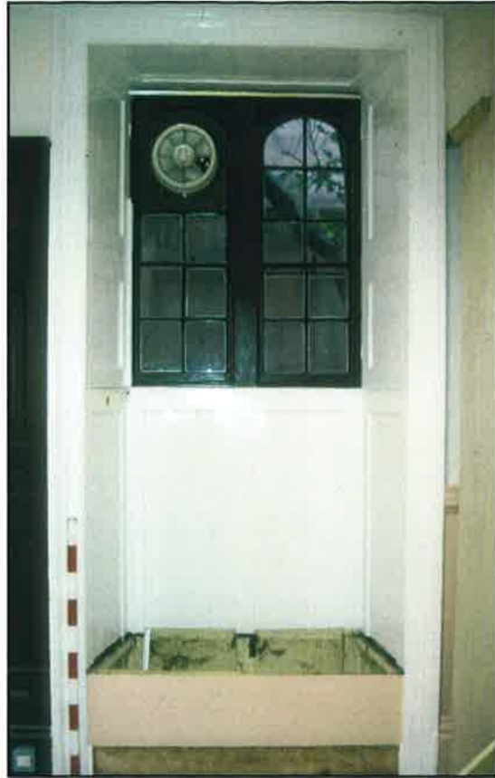
Plate 4: Internal view of window, west elevation
