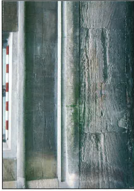
Plate 3: External view of stonework beneath window, west elevation
