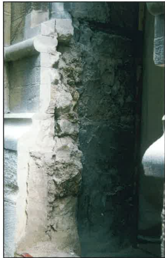
Plate 6: North-east view showing inner core of west elevation
