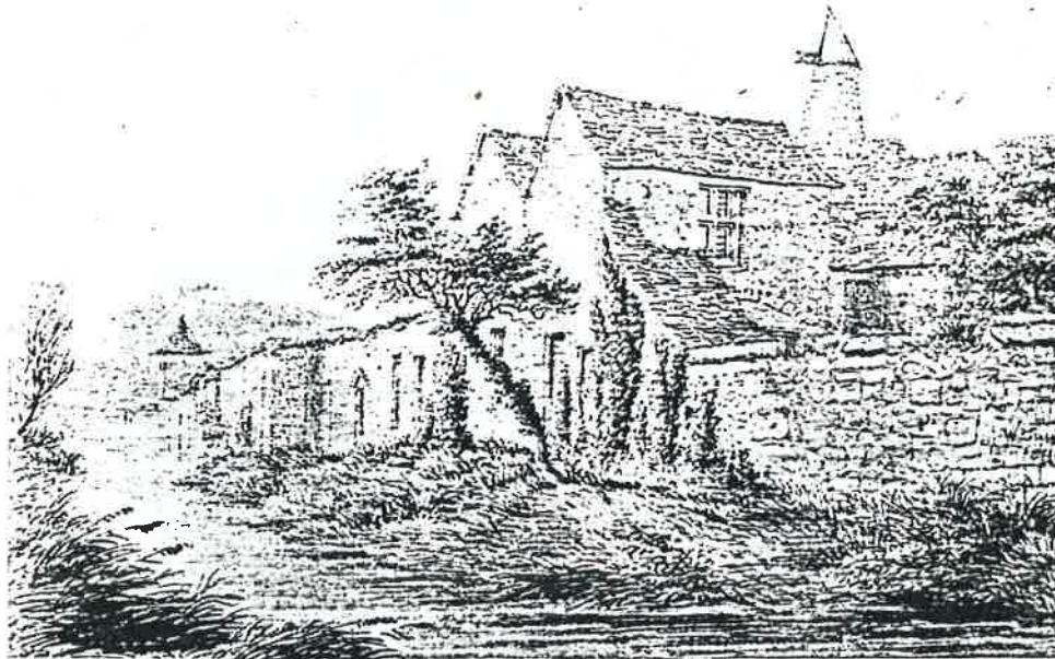
Figure 18B: North range and north-west corner, seen from beyond the moat. Drawing by W. Turner, 1851
