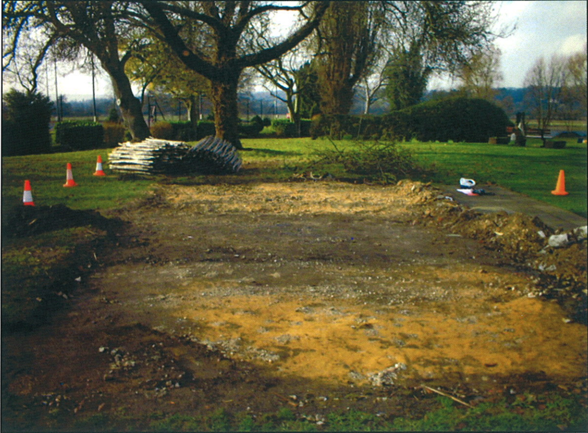
Plate 1: North-west view of Clubhouse foundation area following removal of concrete slab
