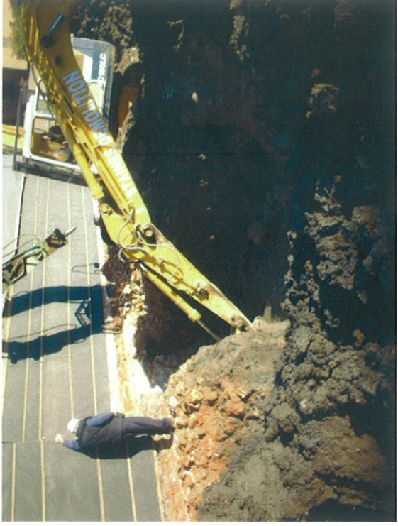
Plate 2: Working shot. Clearing out foundations
