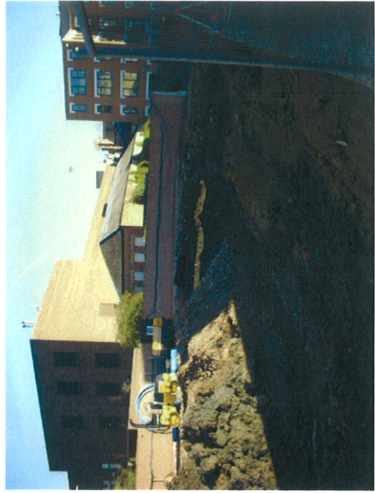
Plate 1: Depth of concrete pads. Pad still remaining in left end of trench
