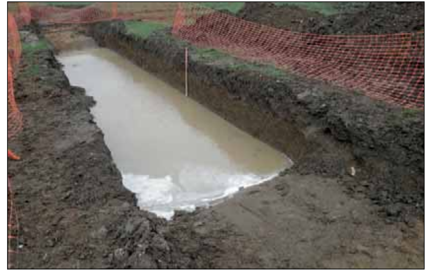
Plate 6: Trench 38, view from east. Pond 135
