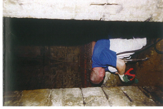
Plate 6: Excavation inside the well chamber
