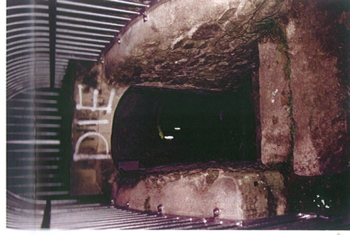
Plate 8: Finished lighting and gate
