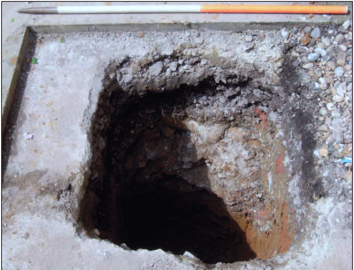
Plate 2: Section 101 looking North-West
