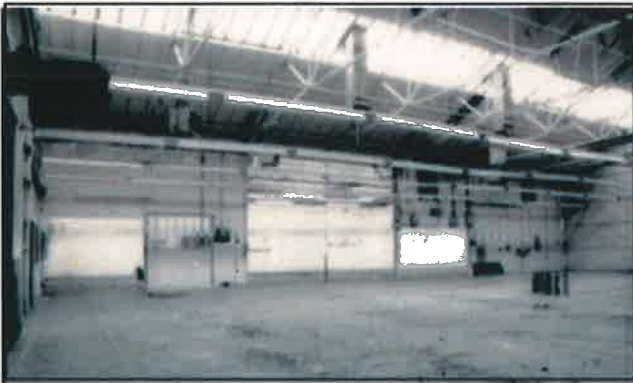
Plate 45: Structural break in the north wall of area 6 (from the south-west)
