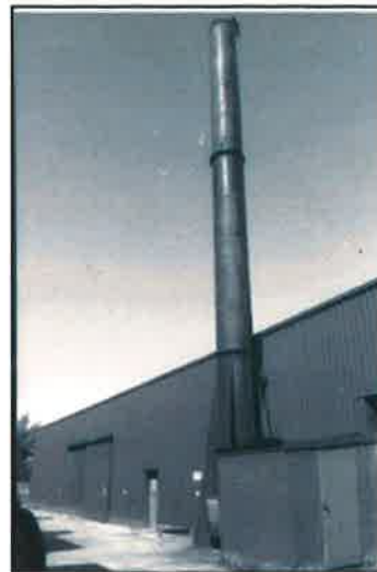
Plate 36: South elevation, chimney (from the south)
