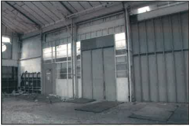
Plate 49: The western end of the area 10/ area 13 partition, detailing the formerly external windows
