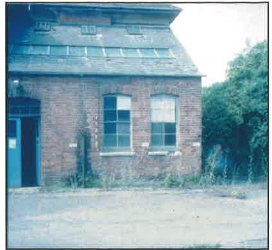
Plate 2: The Extension to the Drinkwater Building (from the east)
