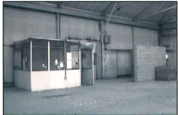
Plate 46: Area 7, north wall, showing office unit and brick partition (from the south-west)
