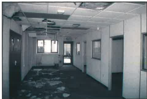
Plate 40: The office area, room 1.1, with double doors the office area 4 on the right of the picture
