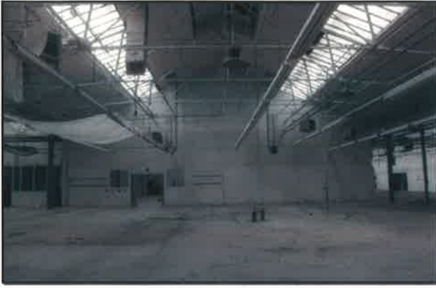
Plate 43: Area 5 looking west, note apex roof and open plan through room 1 (to left) and 9 (to right)
