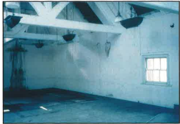
Plate 20: The South-western aspect of room 1/1 (from the north-east)
