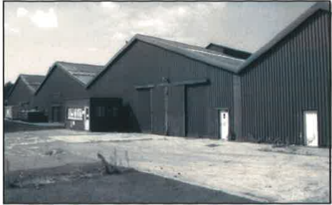
Plate 32: A-shop', aisles 1-3 from the north-east
