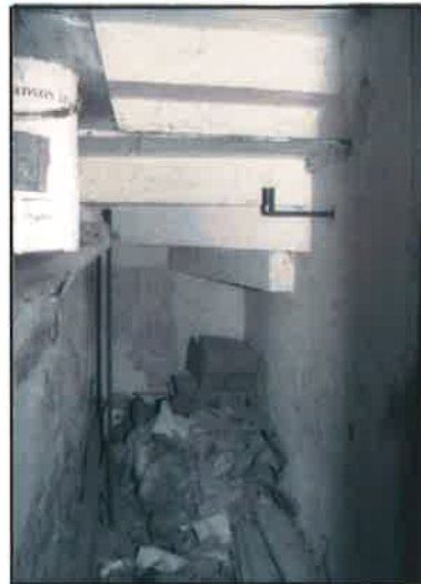
Plate 16: G/3a, the understairs cupboard
