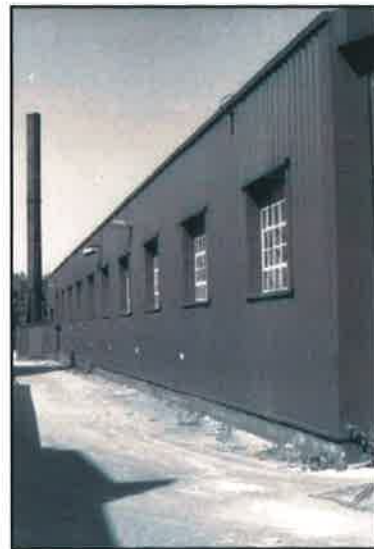
Plate 34: South Elevation showing the windows of room 1 (from the south-east)
