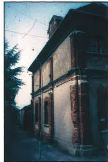
Plate 4: South Elevation showing the damage to brick work and the south chimney (from the south-east)
