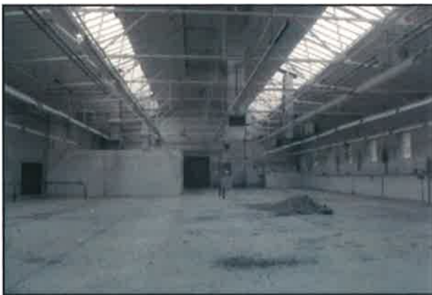
Plate 39: Area 1 looking east
