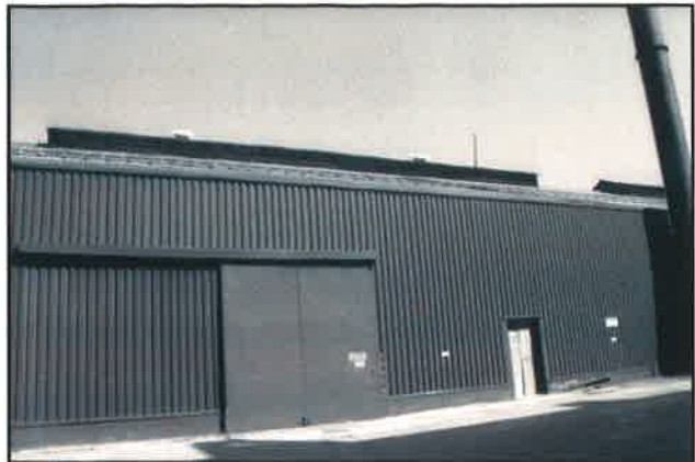
Plate 38: Western half of the south elevation (from the south west)
