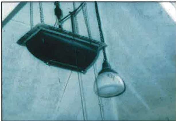
Plate 23: Early 20th century gas fittings
