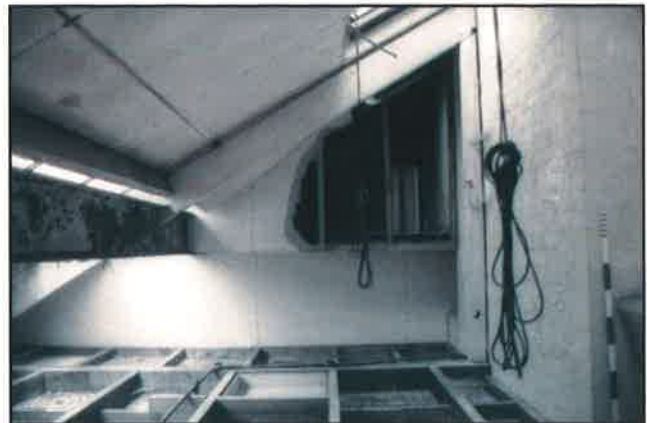
Plate 28: 1/5 looking south, showing exposed floor beams and skylights
