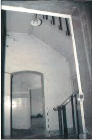
Plate 13: G/3, the stair area looking north
