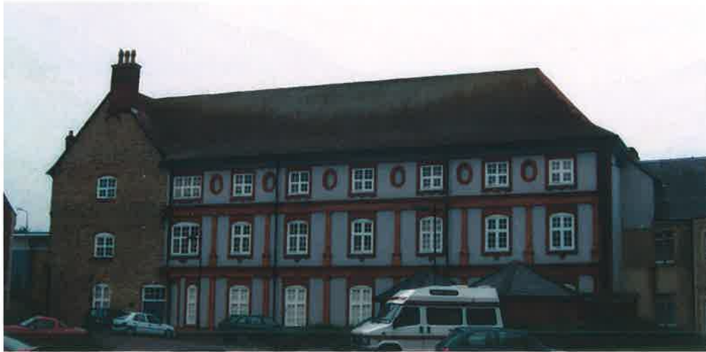
Photograph 1 - The East Wing 1878 (from the south)
