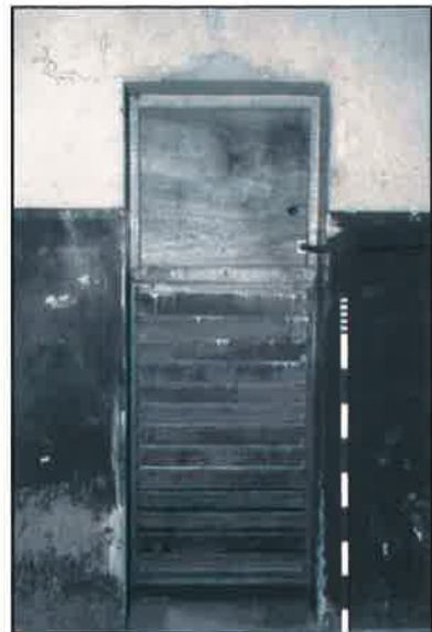
Plate 12: G/6, louvred opening in north wall
