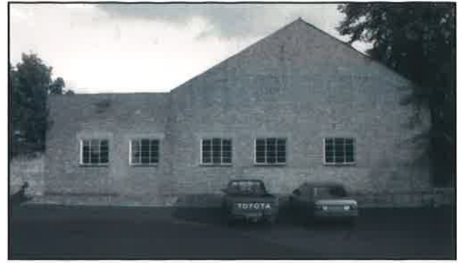
Plate 50: The western elevation of aisle 4 (from the west)
