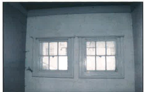
Plate 30: 1/2, east facing windows
