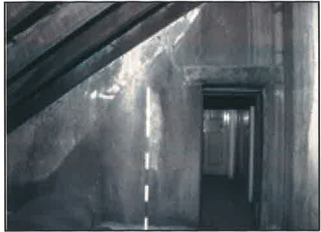
Plate 26: 1/4 looking south, showing half-door and exposed roof beams
