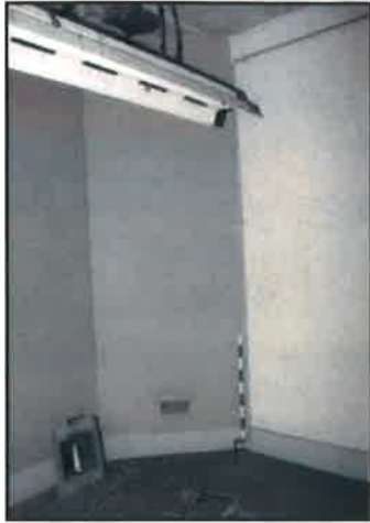
Plate 31: 1/2, chimney in south-west corner
