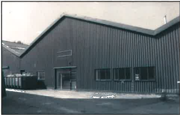
Plate 33: Aisle 3, the office area (from the north-east)
