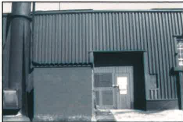
Plate 35: South elevation - chimney, boiler house and external doors (from the south)
