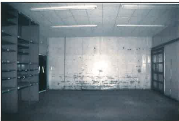
Plate 47: Room 8, north wall showing shelving units down west wall (from south)
