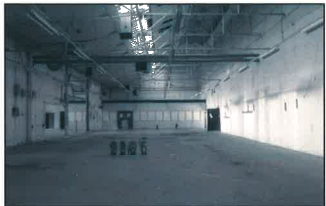
Plate 48: Area 9 from the east, showing office units at the west end and the partition wall to north
