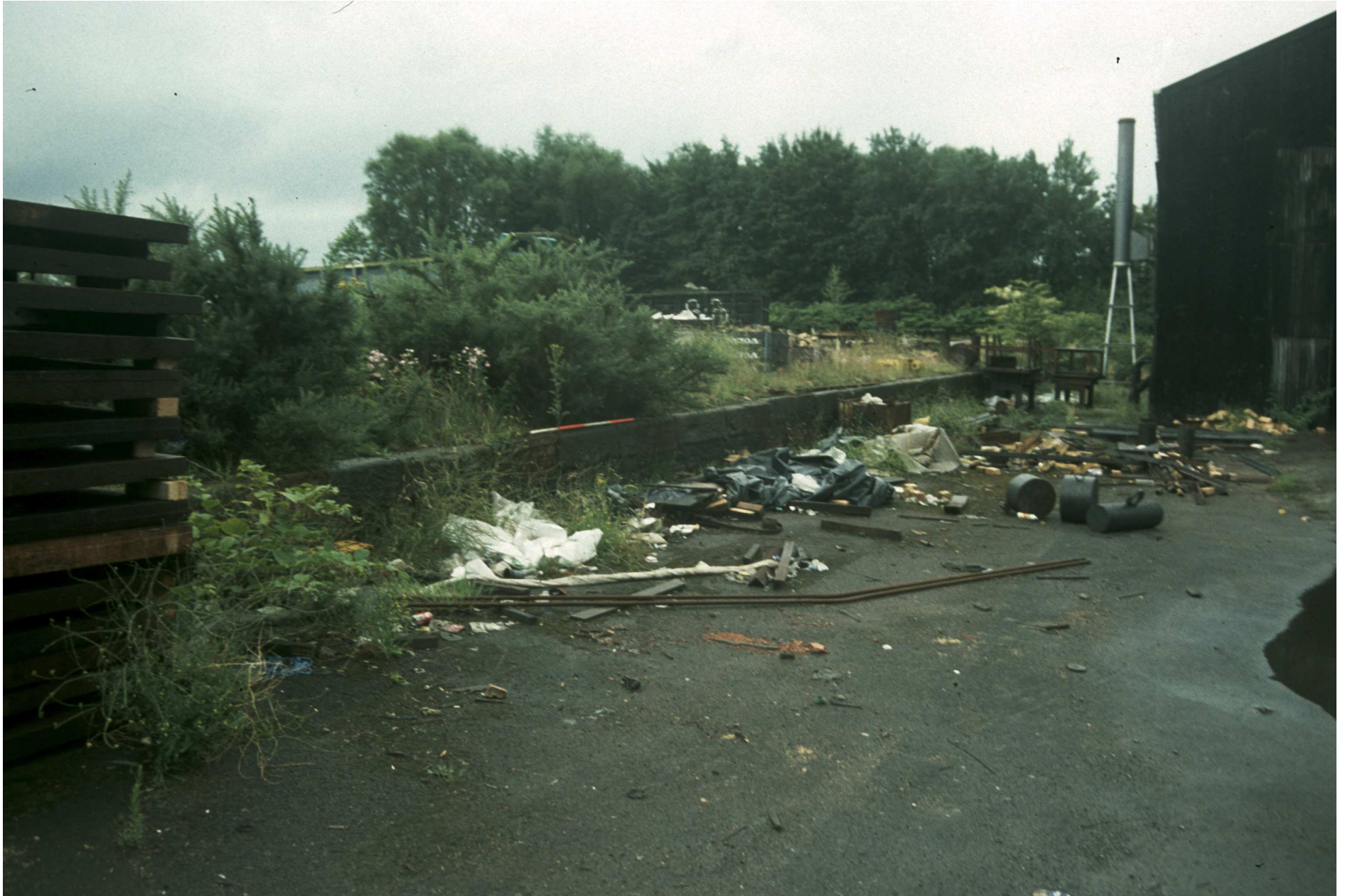
Plate 1: General view south of the North Dock Basin (east side)
