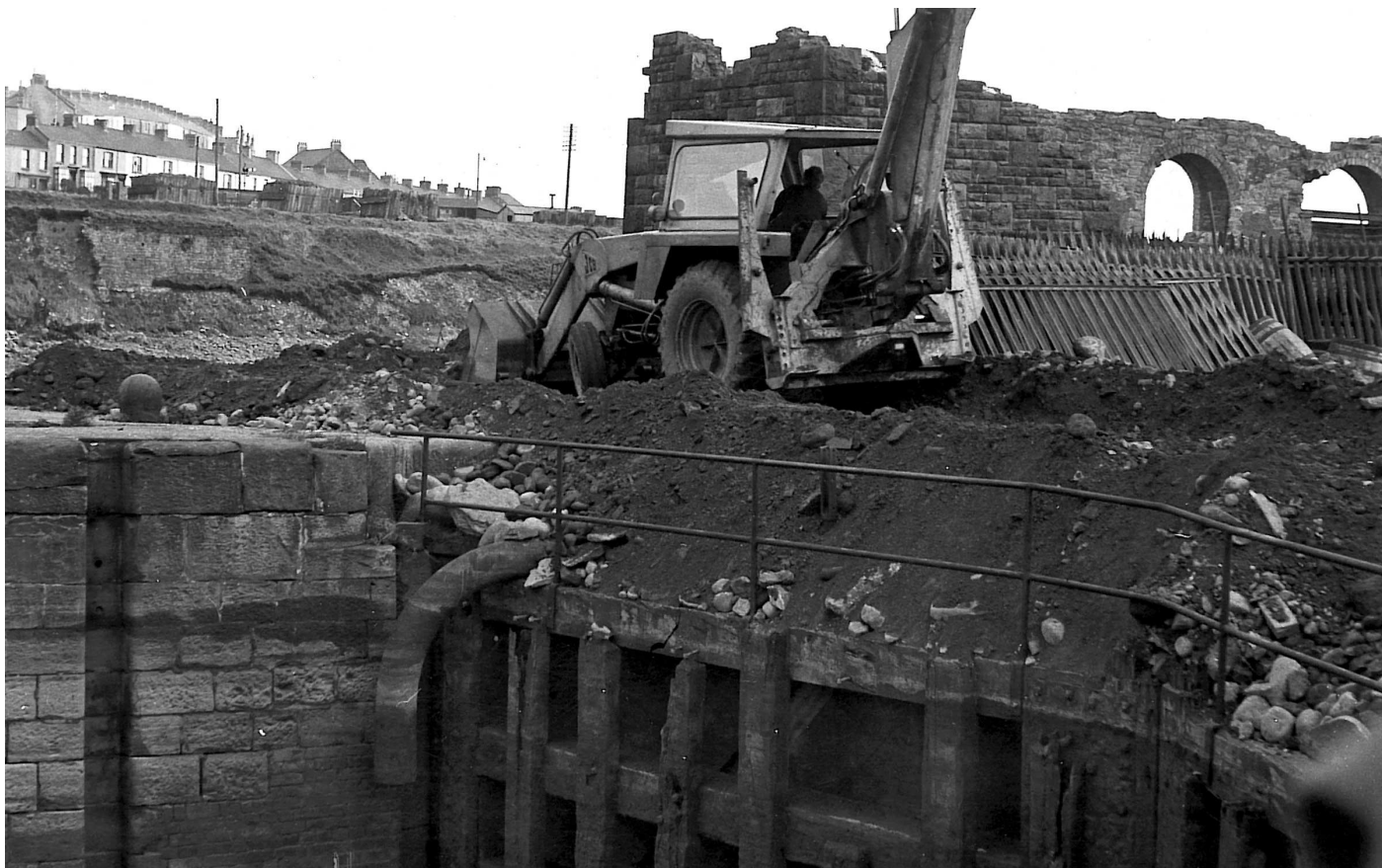
Plate 5: 1965 reclamation and backfilling of the North Dock Basin (courtesy of USE)
