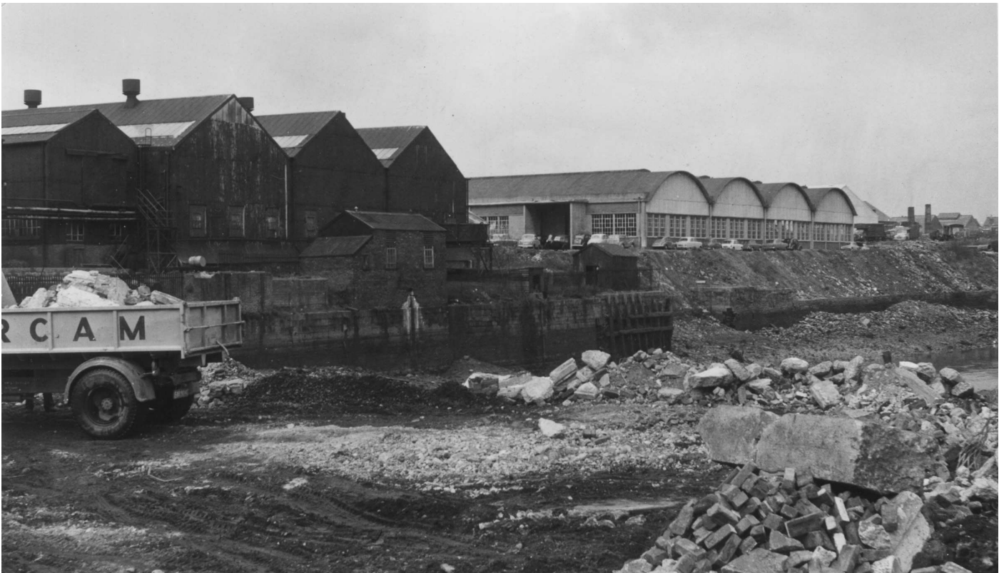
Plate 8: 1965 reclamation view NW with the extant Jersey Dock entrance in the near background (courtesy of USE)
