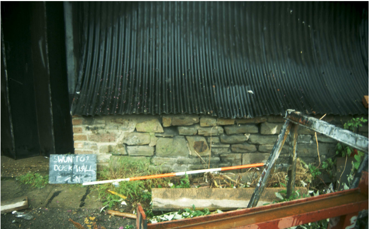
Plate 3: General view of the stone dwarf wall at the eastern end of the factory
