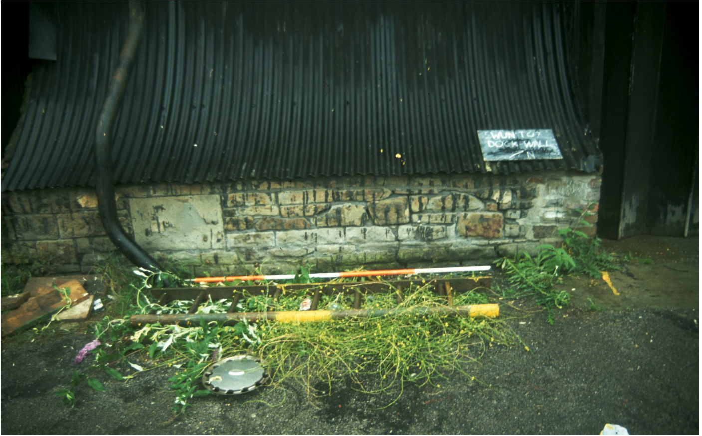
Plate 2: General view of the stone dwarf wall at the eastern end of the factory
