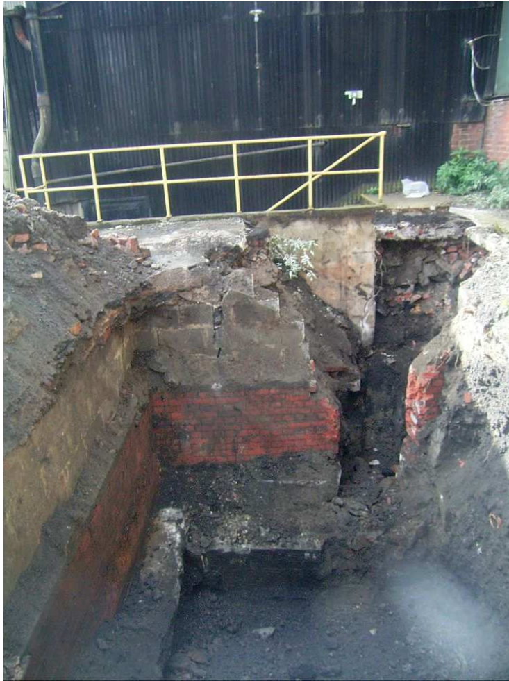
Plate 1. Trial Trench 9/10 showing the dry dock wall beneath a modern brick and block wall. View SSW
